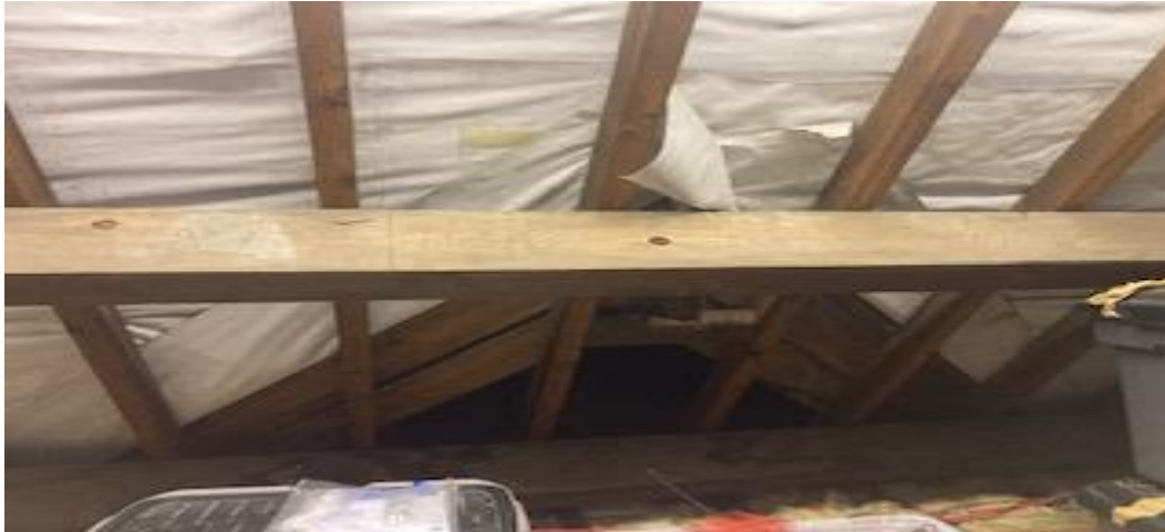
Plate 6 - Internal views of southern wall in loft
