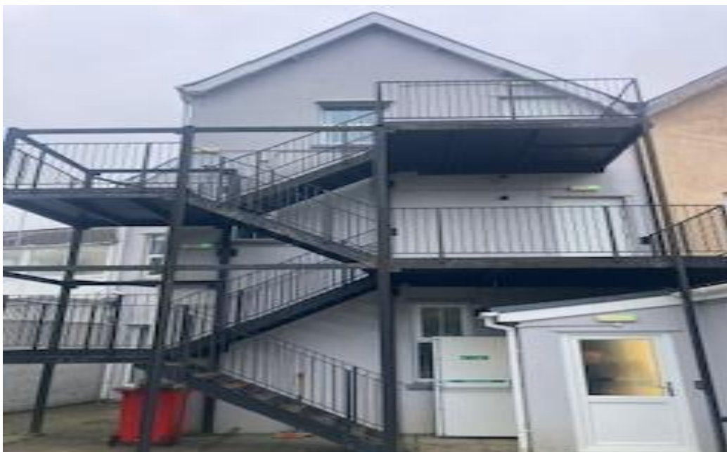
Plate 2 – Western (Rear) elevation
