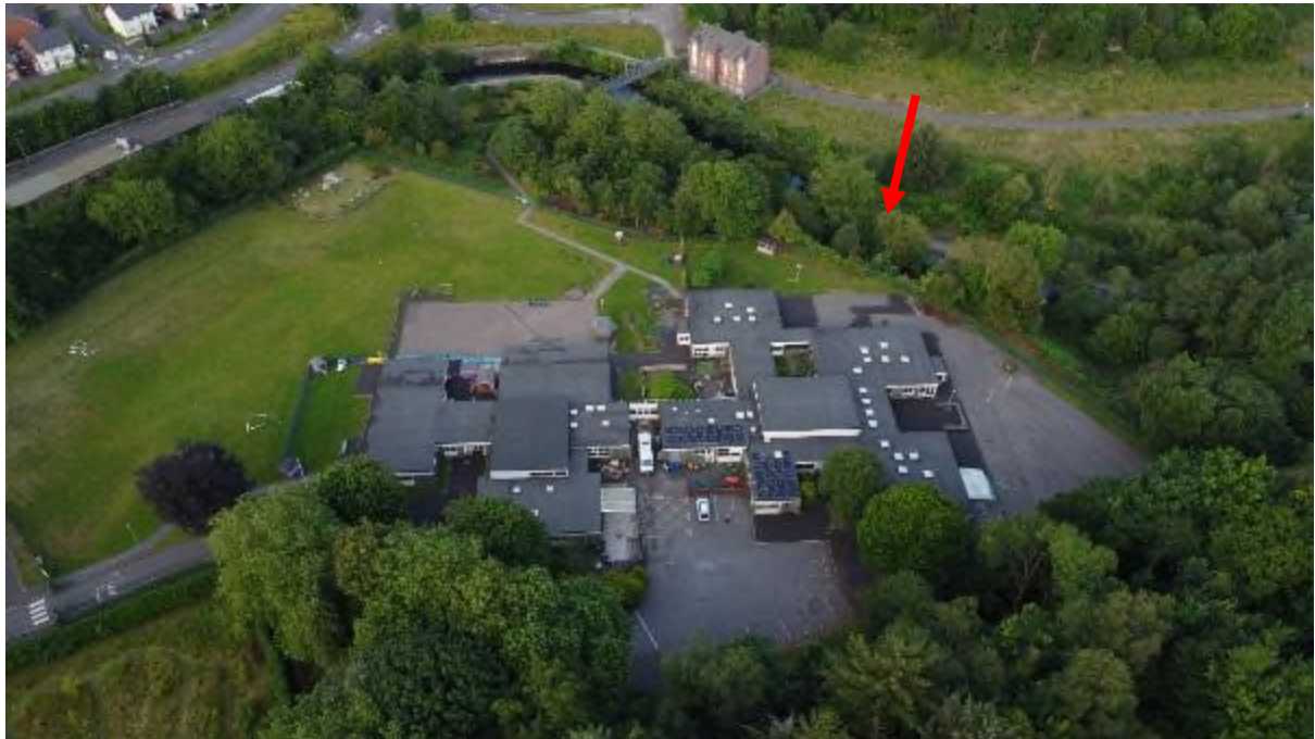
Plate 3 west facing aspect at the side of the school showing location of river Taff
