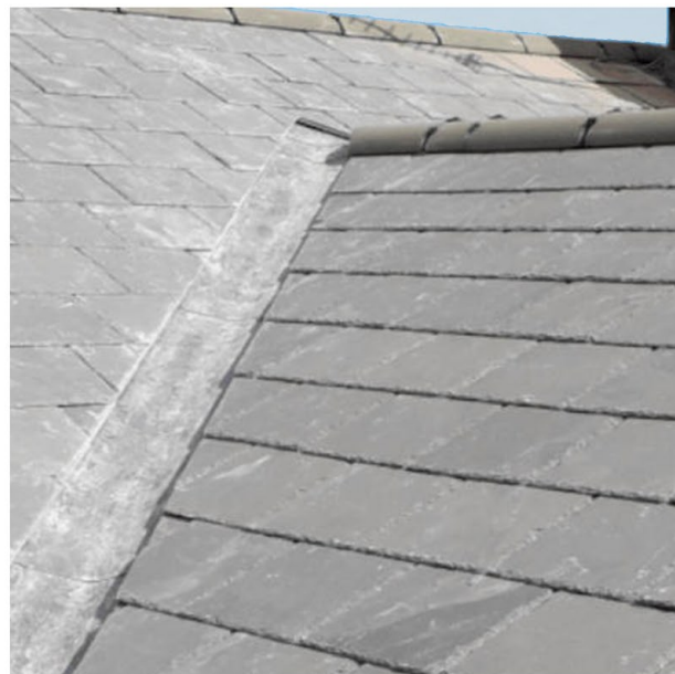
1 Roof: Natural grey slate with matching vented ridge tiles
