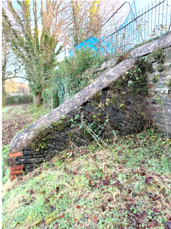
Photograph 11 : View of left stone buttress (right side).
