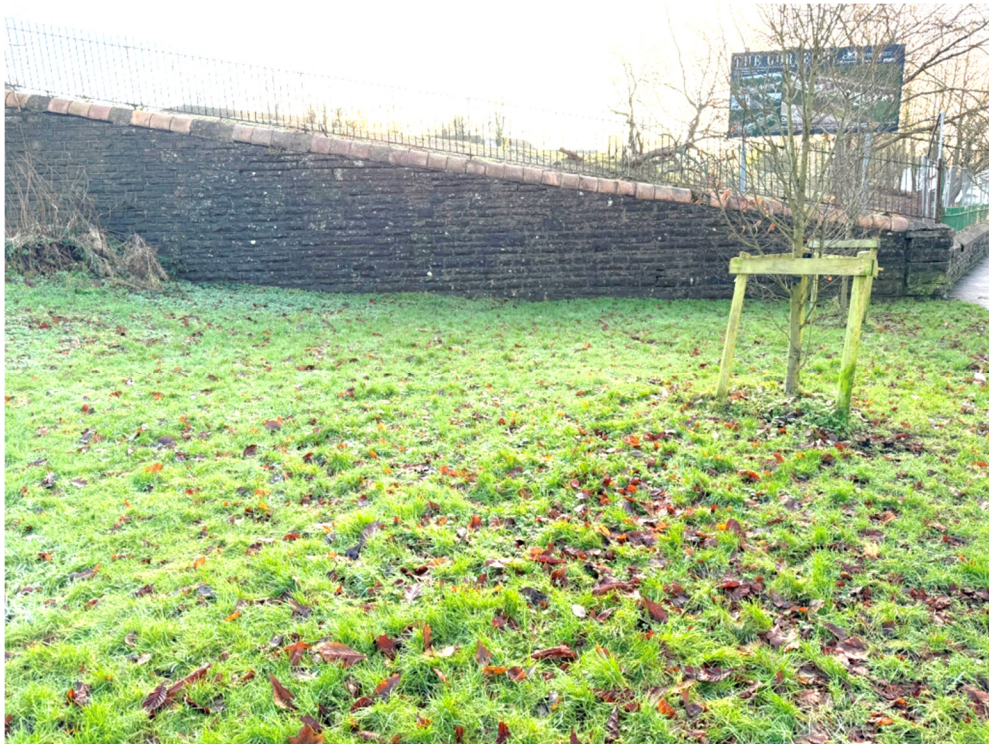
Photograph 4 : View of right hand length of retaining wall with diminishing retained height.
