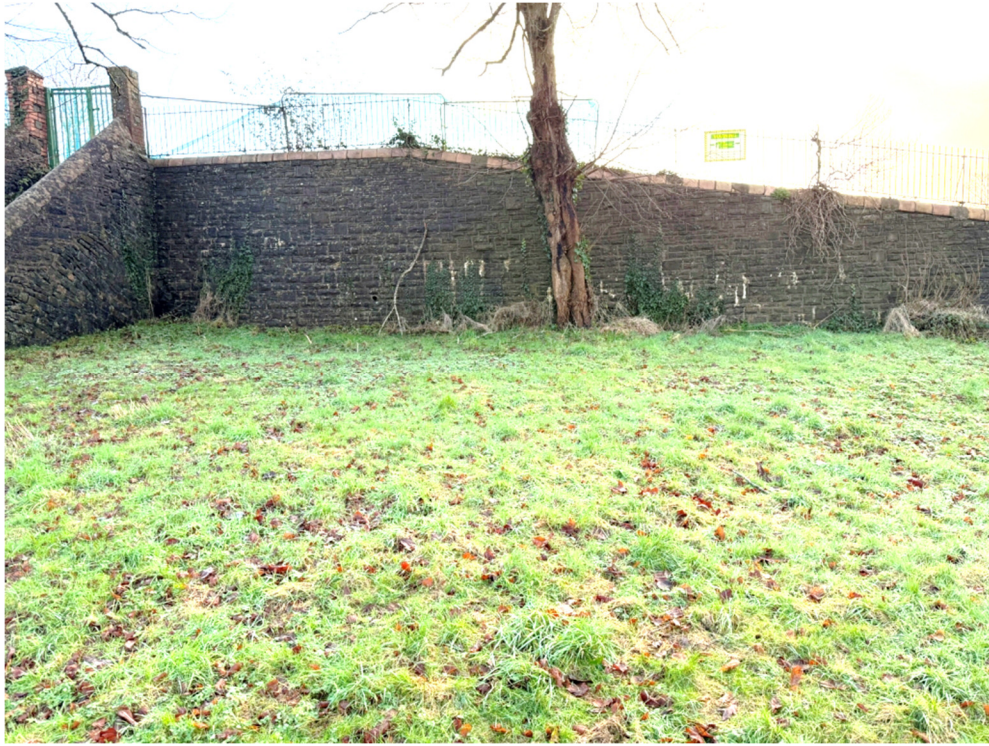
Photograph 3 : View of random stone boundary retaining wall to right of access steps
