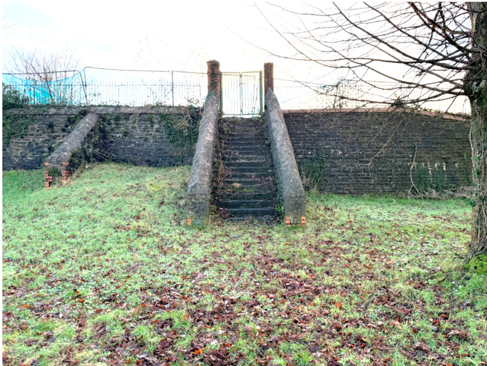
Photograph 2: View of access steps and stone buttress adjacent retaining wall.
