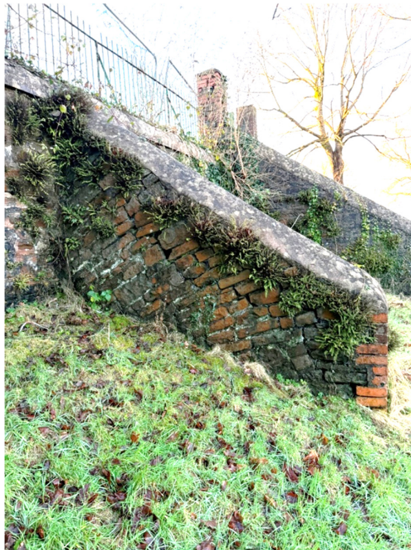
Photograph 10: View of left stone buttress (left side).
