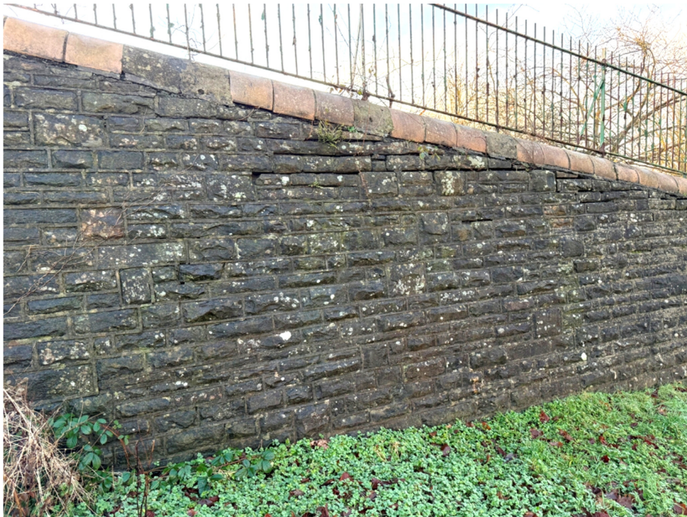
Photograph 20: Another view of right hand length of random stone boundary retaining wall. Retaining wall along this length appears in a stable condition at the time of or inspection.
