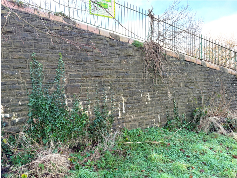
Photograph 19: No other drainage weep holes are provided. Right hand retaining wall appears in a stable condition at the time of our inspection.
