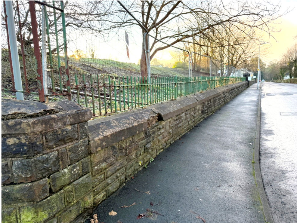
Photograph 23: View of small front retaining wall along Queens Road.
