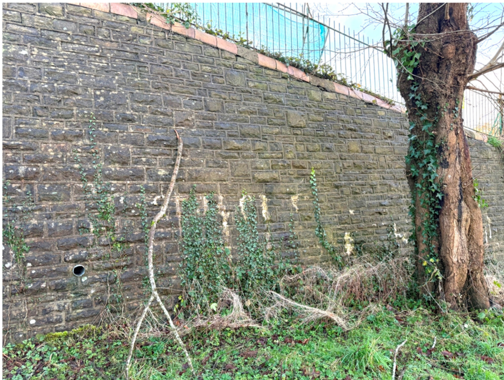
Photograph 18: 2no. drainage weep holes are evident just to the right of the access steps. No evidence of damaged to the retaining wall from tree roots.
