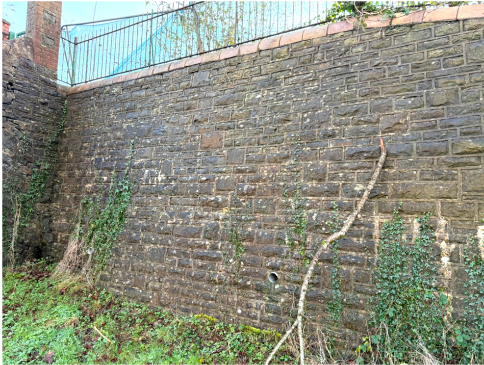
Photograph 17: Retaining wall is approximately 3.50m high at its maximum. Right side retaining wall appears structurally stable with no sign of cracking, open jointing or lateral distortion.
