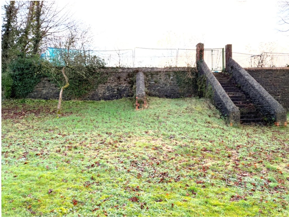
Photograph 1: View of random stone boundary retaining wall to left of access steps.
