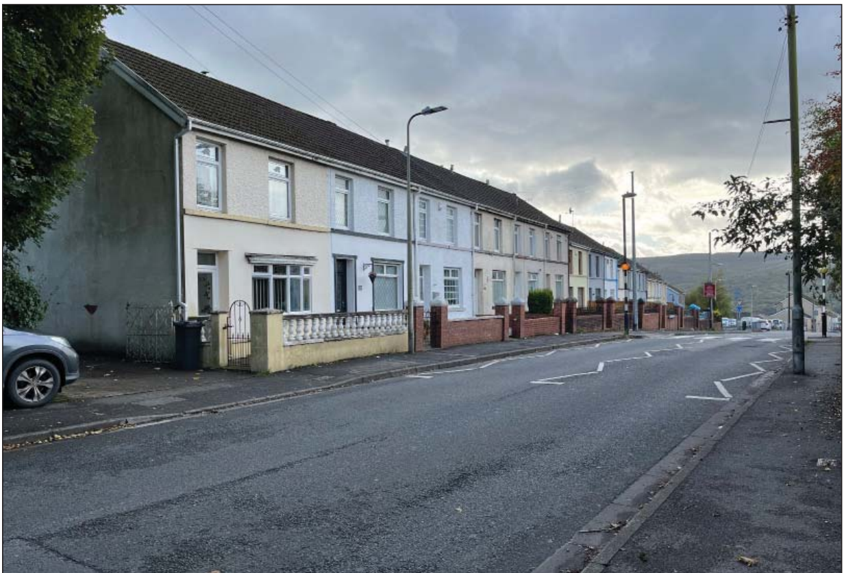
Plate 12 - View of Merthyr Tydfil: Historic and Commercial Core (HCLA 001) beyond the northern corner of Site, looking southwest
