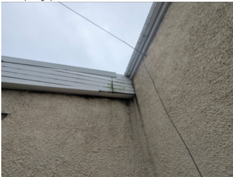
Plate 2- photograph of sealed fascias and soffits
