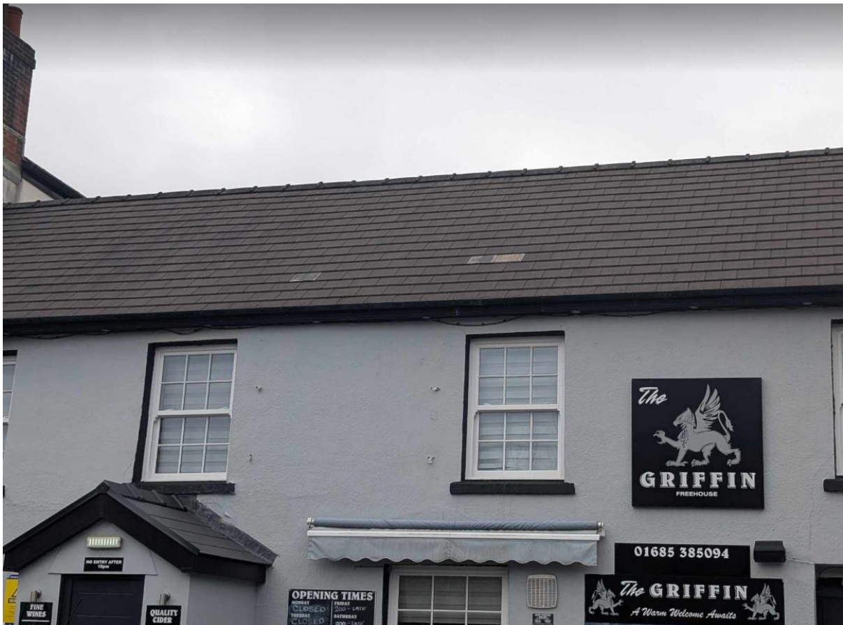
Plate 2- photograph of tight fitting slates on front elevation
