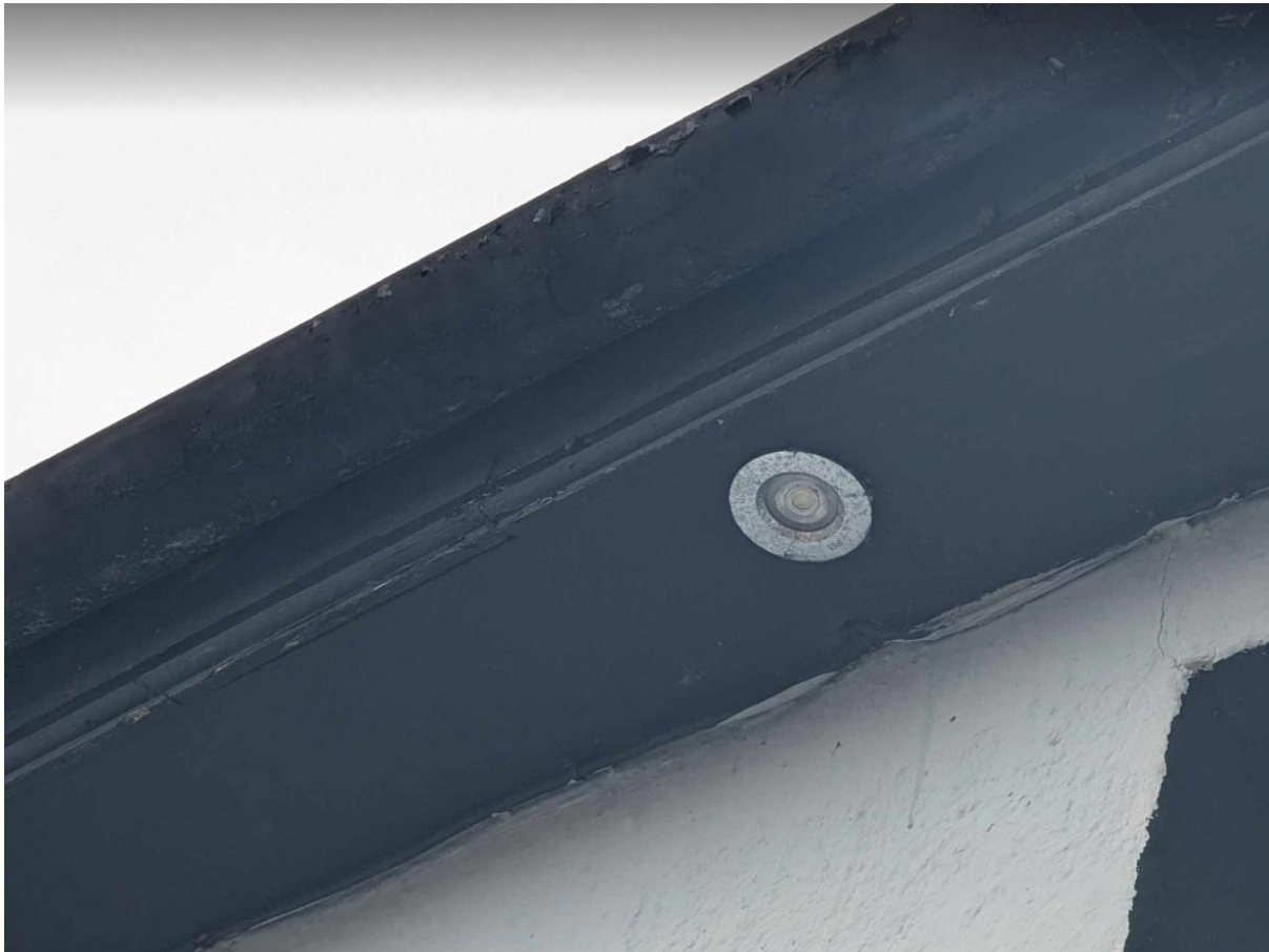
Plate 6- tight fitting soffits
