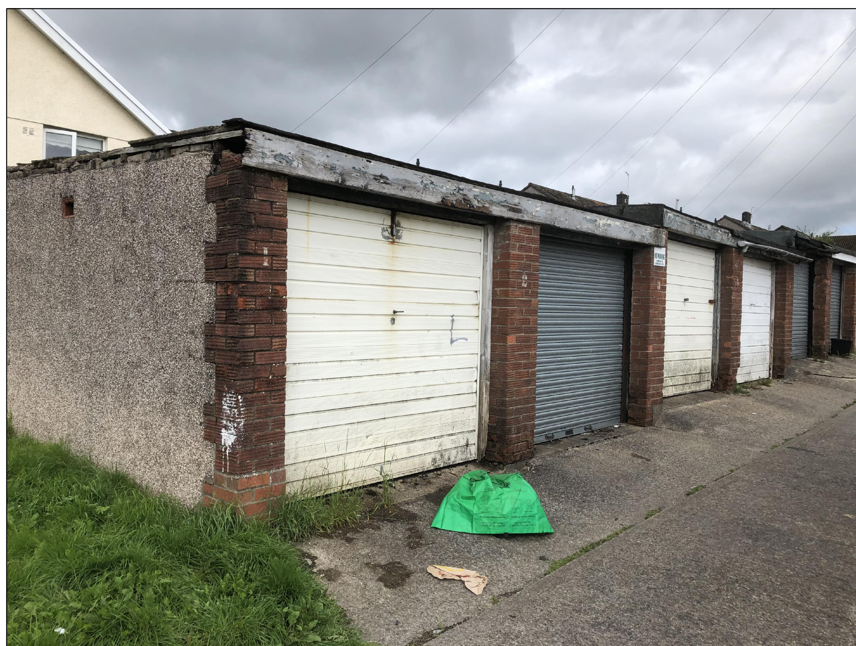
Photo of the existing garages
