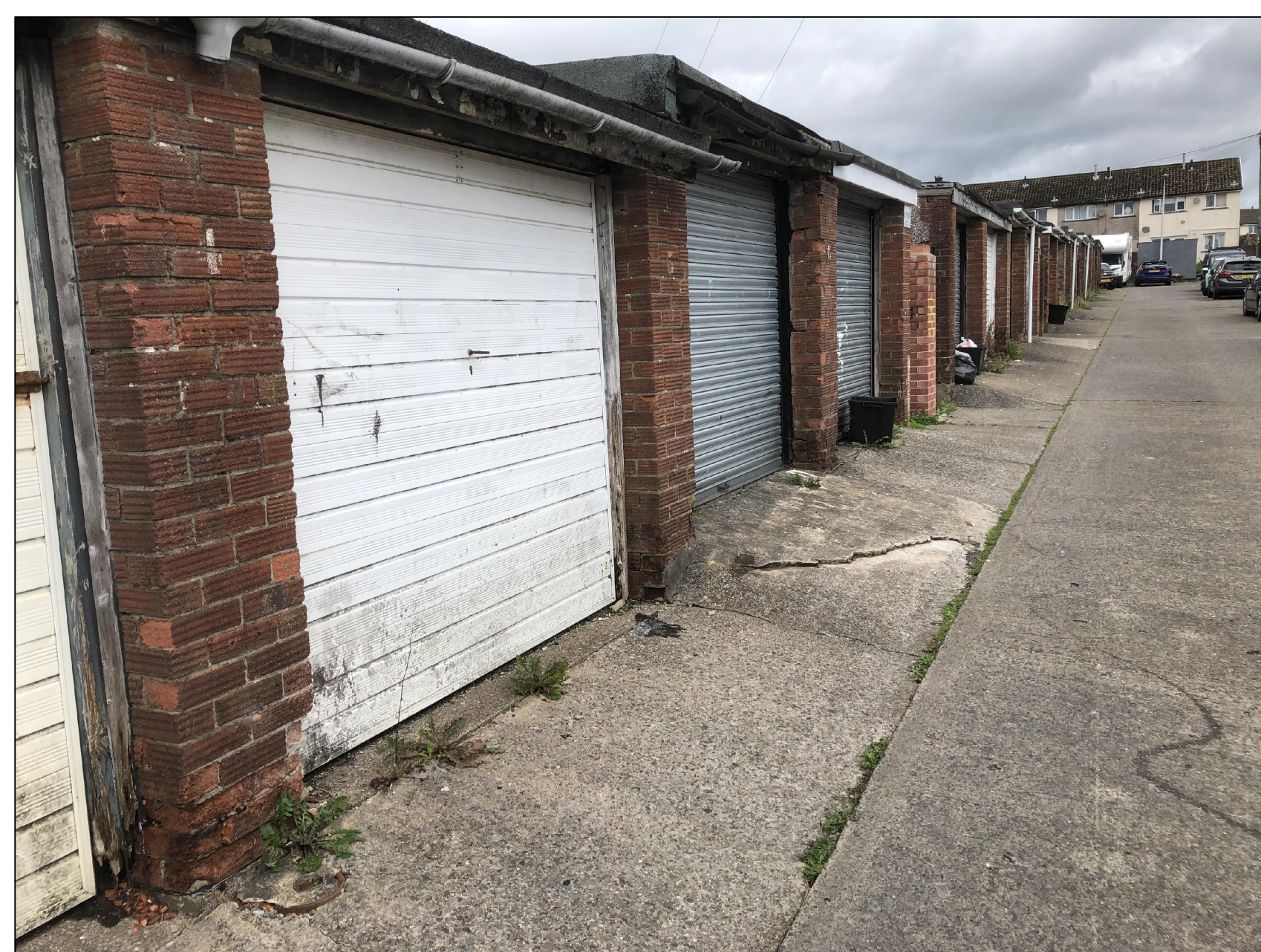
Photo up Pine Close of the existing garages
