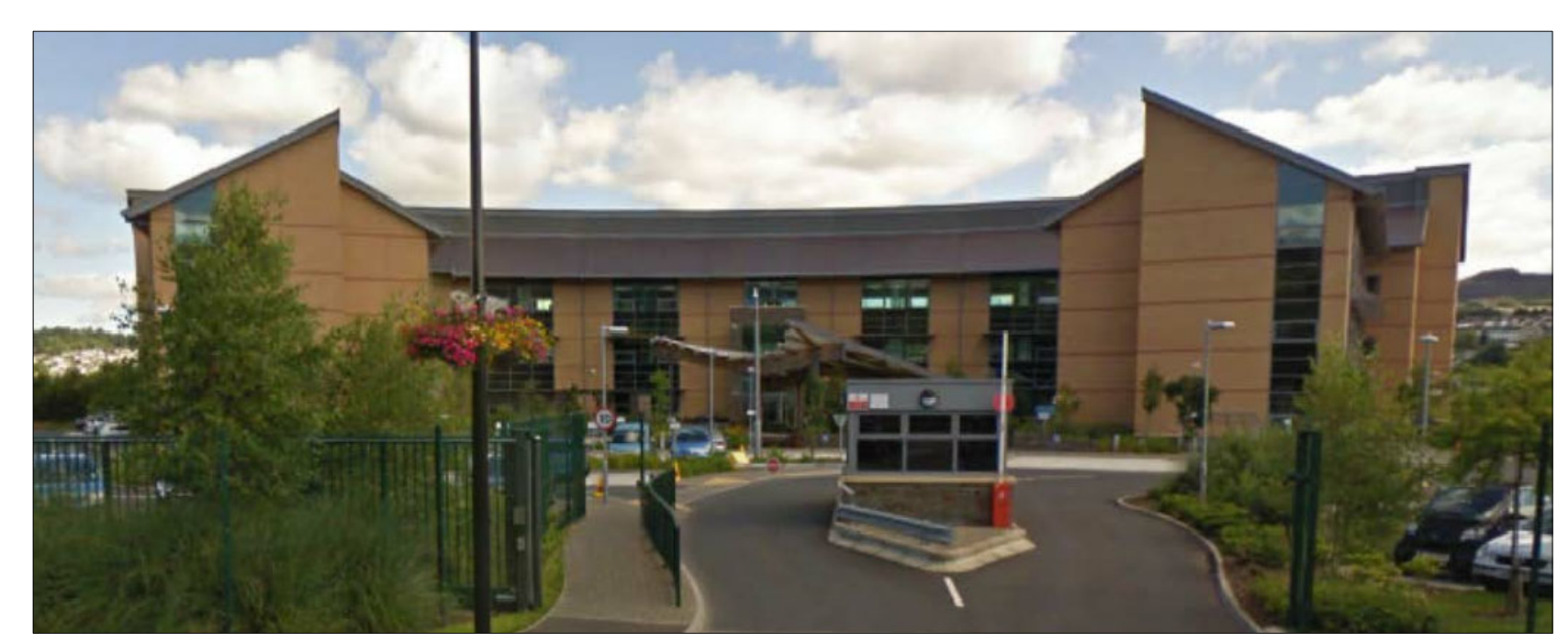
05 EXISTING BUILDING PHOTOS
