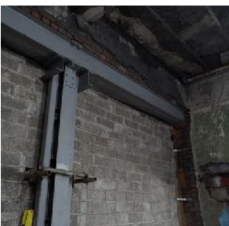
Below left and below: The ground floor steelwork supporting the Front Building, eastern colonnade:
