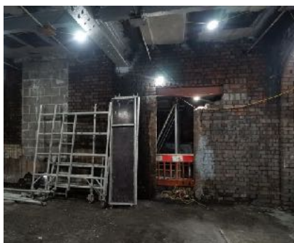
Left: Various internal repairs and alterations:
