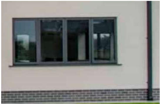
Anthracite grey windows, RWG & engineering brick plinth
