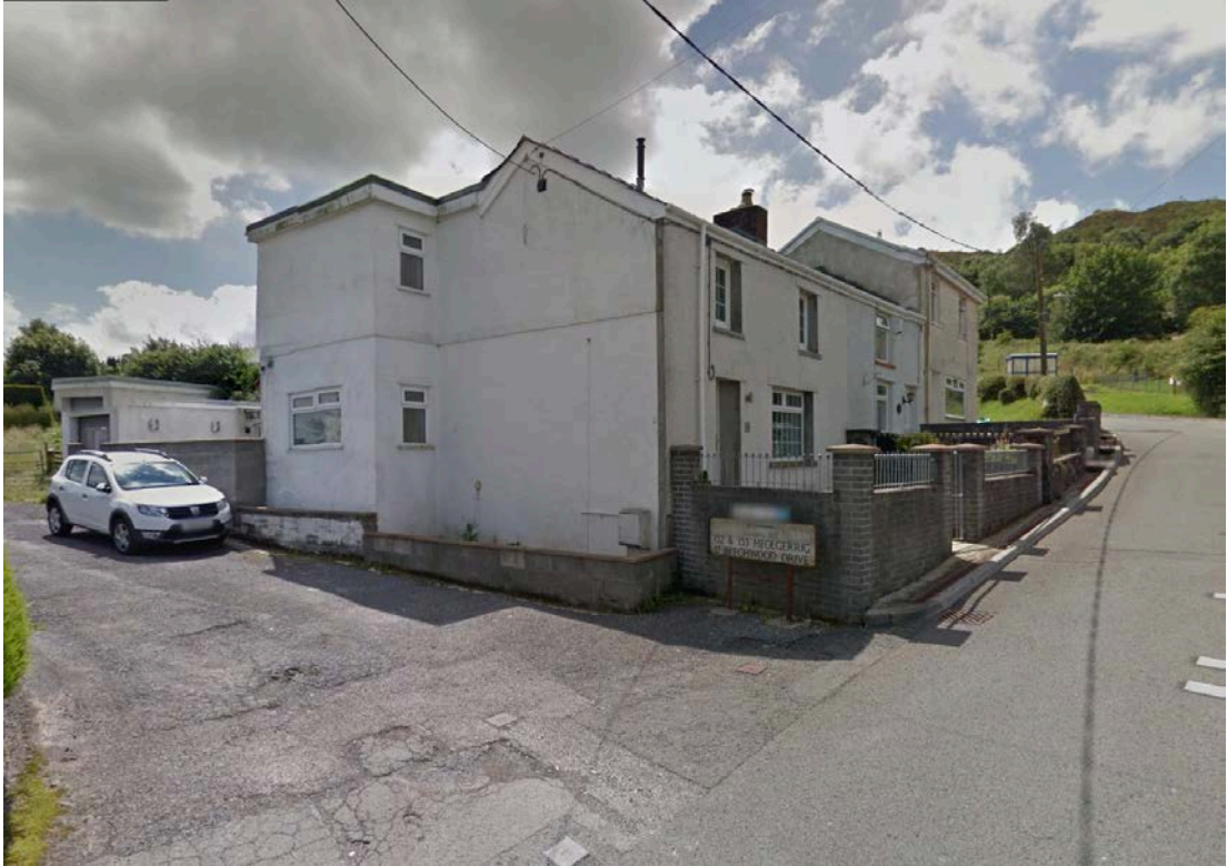
Heolgerrig Junction / Access
