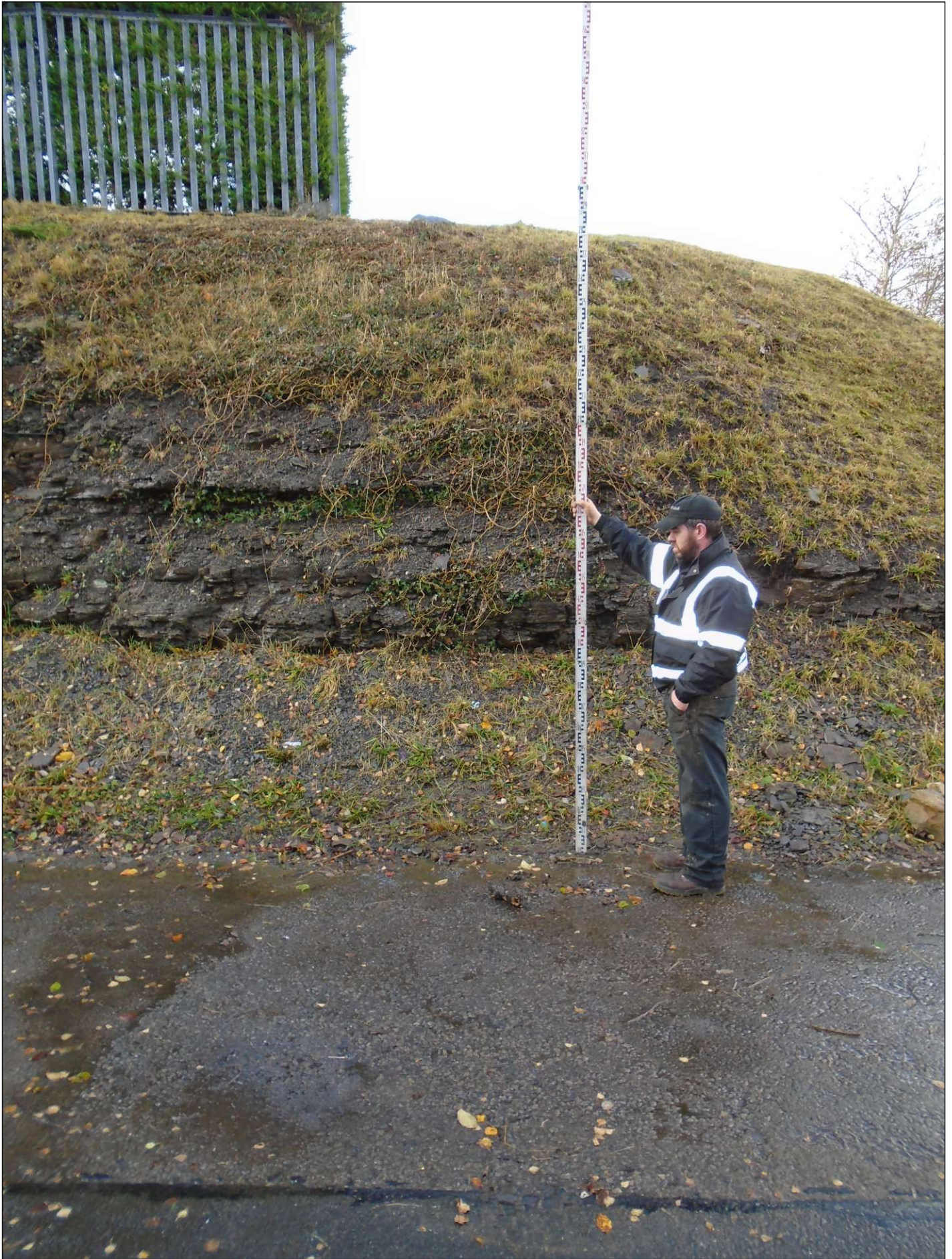
FIGURE 4 WITH THE STAFF HELD VERTICALLY THE TOP OF THE EMBANKMENT AT THE CORNER OF THE PALLISADE FENCE WAS APPROXIMATELY 4.2m ABOVE THE YARD LEVEL
