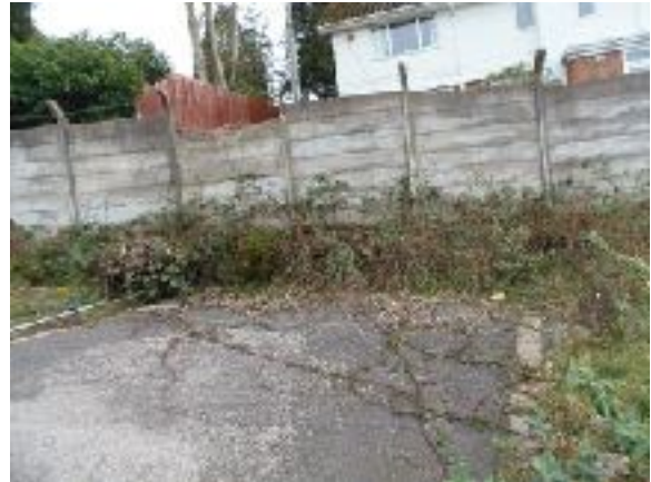
Turning head in north east of site
