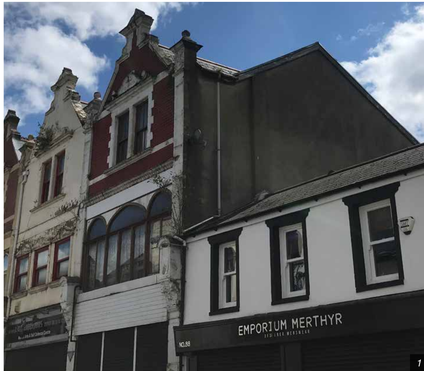
1 Morlais Buildings, High Street, Merthyr Tydfil
