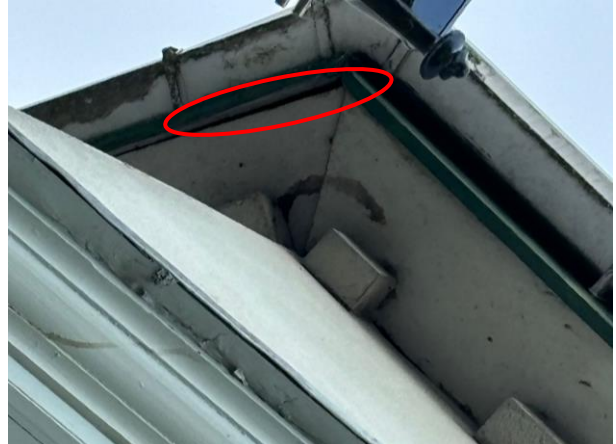
Photo 18: Lifted Lead Flashing North-Eastern Elevation (Circled)
