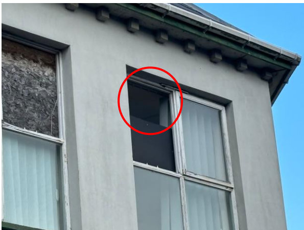
Photo 11: Partially Boarded Window on First Floor of Southern Elevation (Circled)
