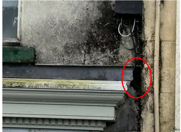
Photo 18: Lifted Lead Flashing North-Eastern Elevation (Circled)
