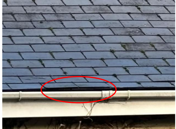
Photo 10: Gap Between The Soffits on South-Western Elevation (Circled)
