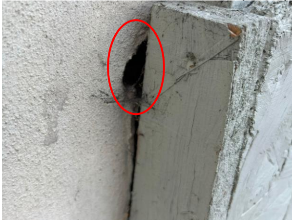
Photo 17: Gap Between Decorative Timber and External Wall on North-Eastern Elevation (Circled)
