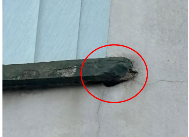
Photo 16: Fascia Lifted from Soffit on Eastern Elevation (Circled)
