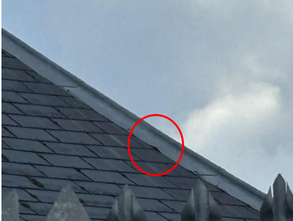
Photo 9: Gap Under Ridge Tile (Circled)
