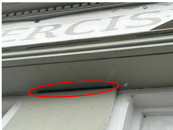
Photo 22: Gap in Decorative Timber on North-Eastern Elevation (Circled)
