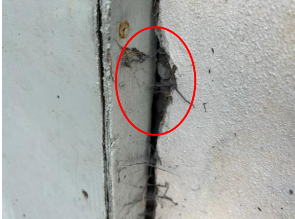
Photo 17: Gap Between Decorative Timber and External Wall on North-Eastern Elevation (Circled)
