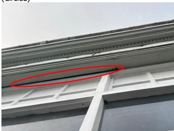
Photo 21: Gap Between Decorative Timber and Timber Window Frames on North-Eastern Elevation (Circled)
