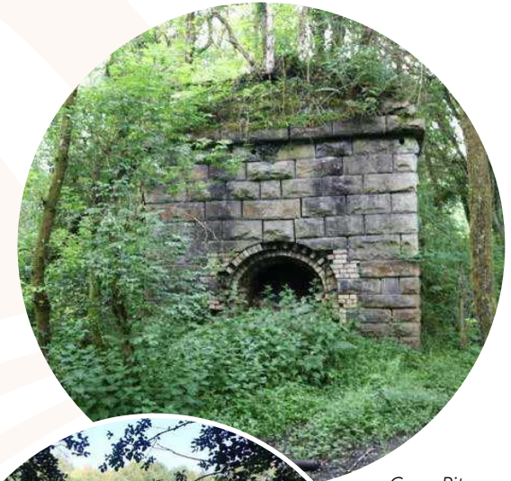
Cwm Pit Chimney Base
