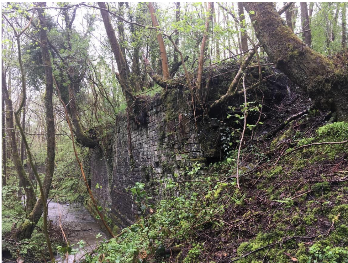
Fig. 1. General view of the retaining wall (20/05/21)
