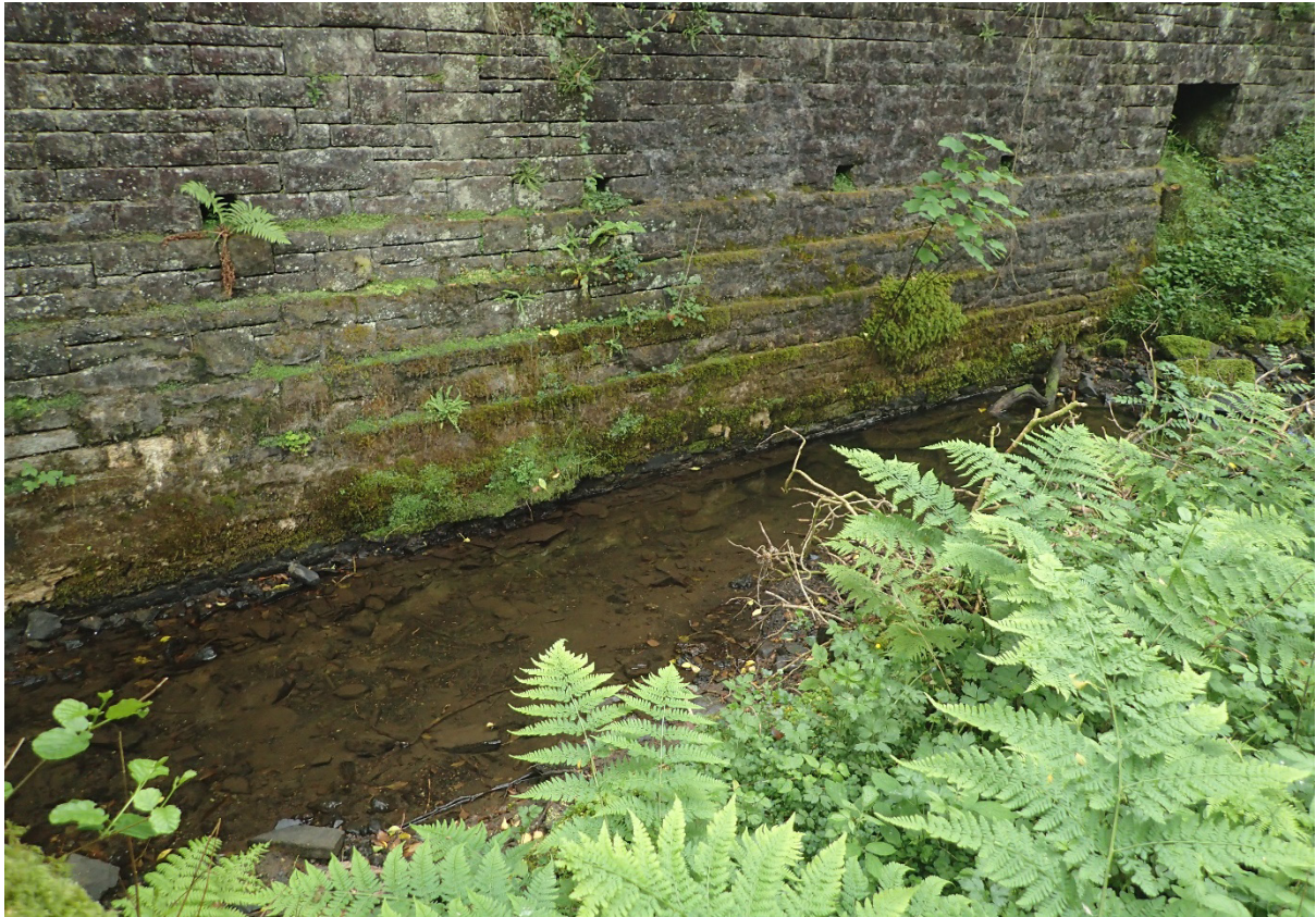
Image EDP 15: Image showing the water course at Cwm Pit running directly past the revetment wall.
