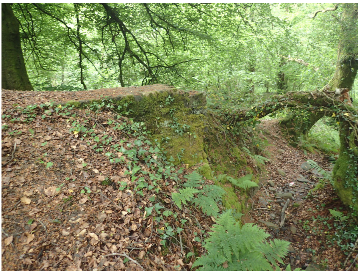
Image EDP 11: Brickwork preserved at one of the sluices at the Pond and Leat.
