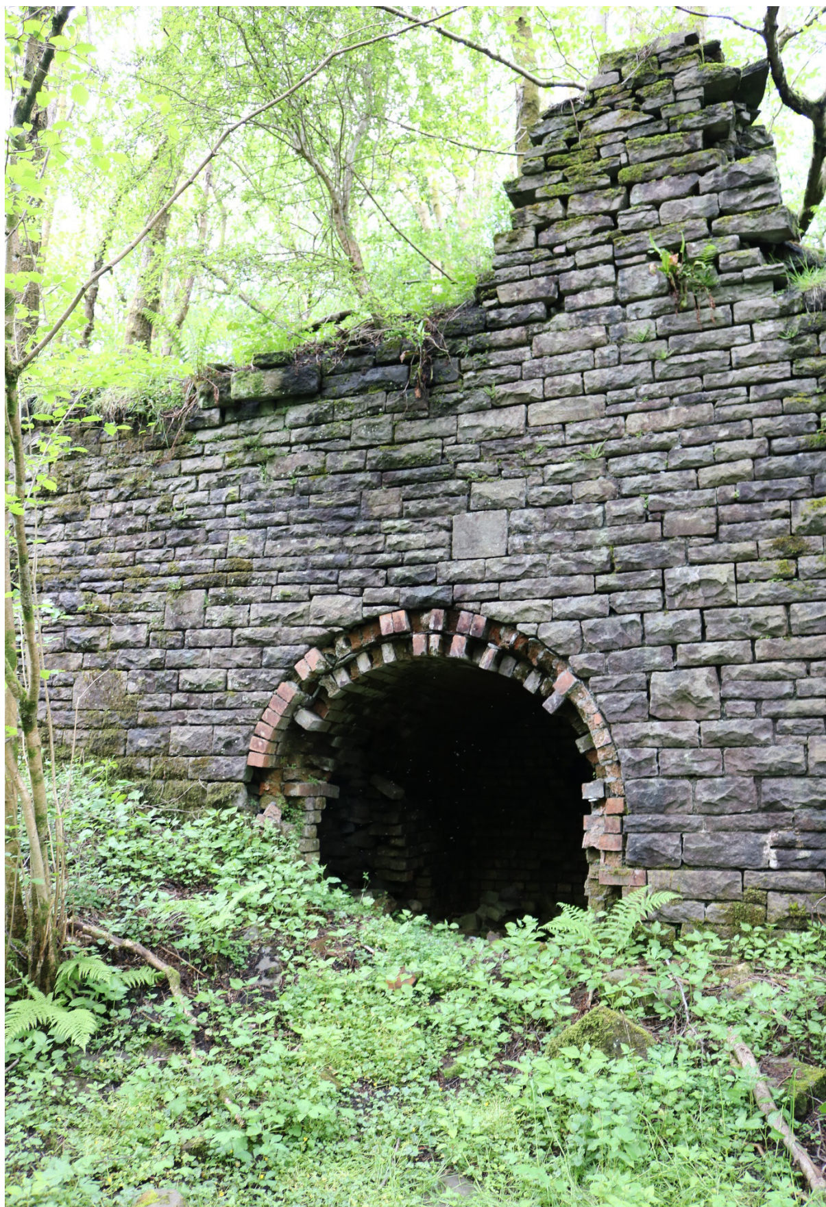
Image EDP 4: The northern wall section at Cwm Pit.
