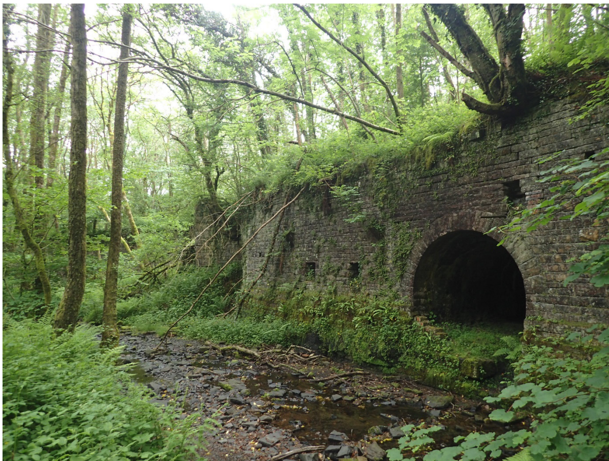
Image EDP 5: The south-western part of the massive stone revetment wall at Cwm Pit.
