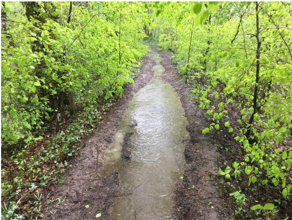
Fig. 3. Erosion to pond/leat top of earthwork bank & standing water (20/05/21)
