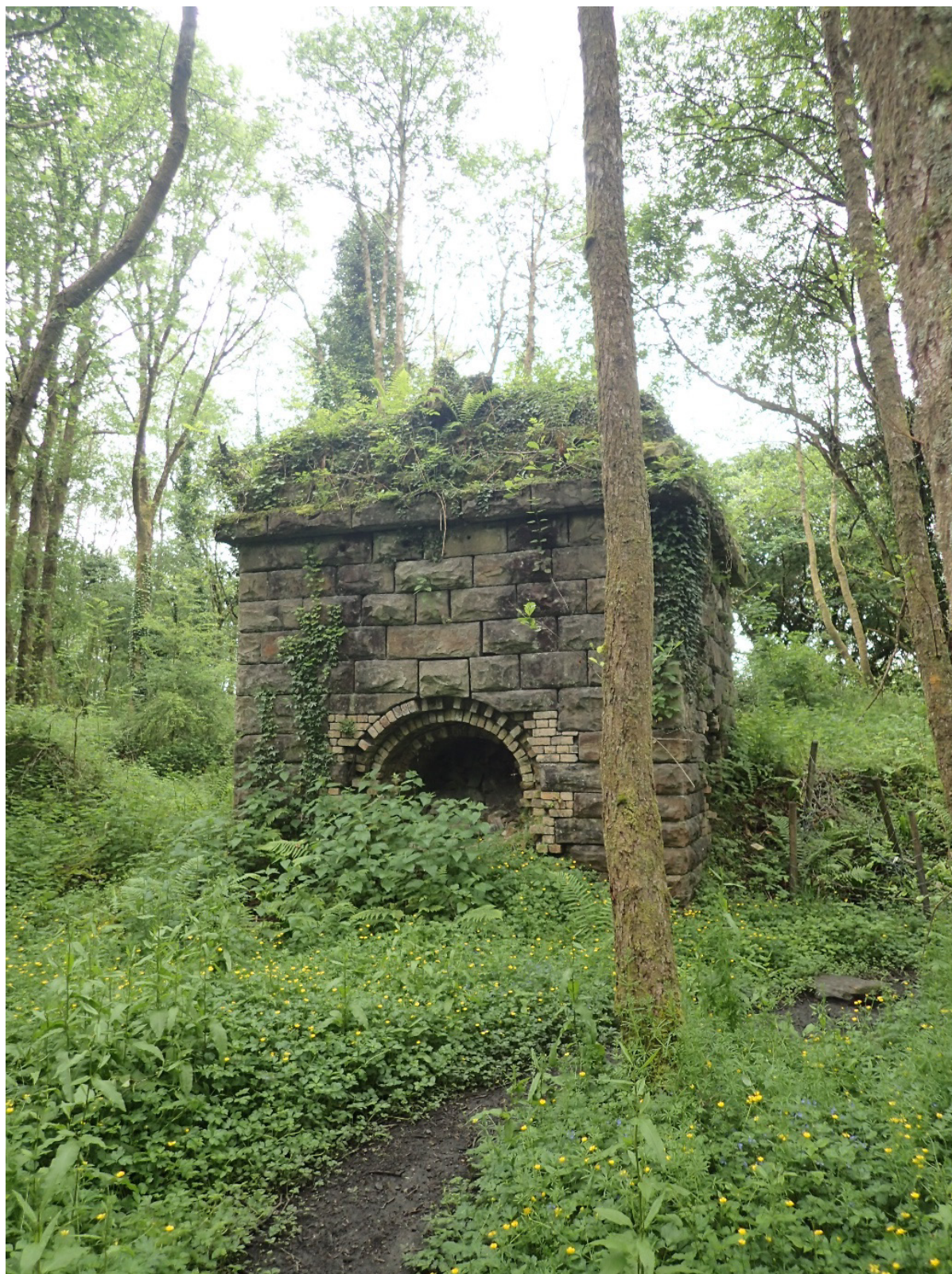
Image EDP 6: The Grade II listed chimney base at Cwm Pit.
