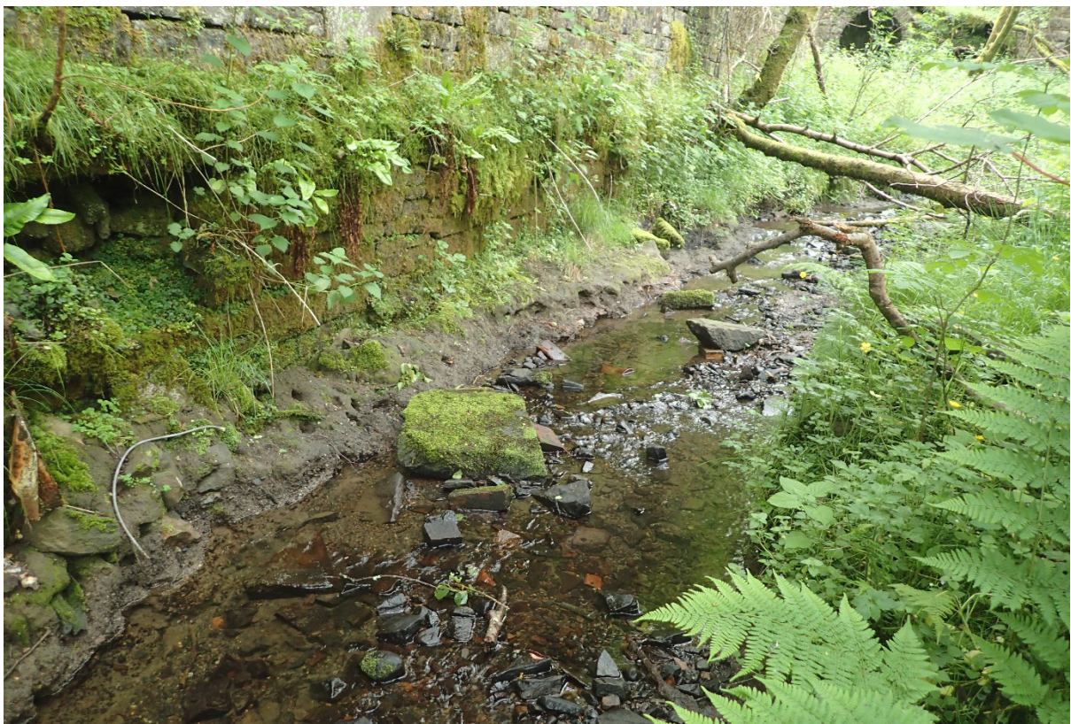
Image EDP 16: Image showing the water course at Cwm Pit running directly past the revetment wall.
