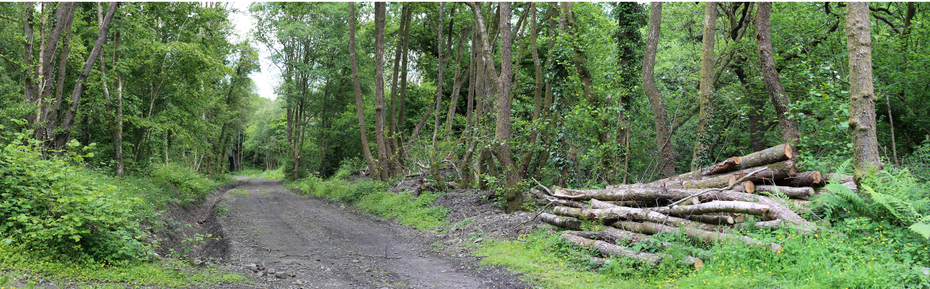
al area of the site showing the recent engineering works that have been carried out by Merthyr Council showing the construction of a drainage ditch, the removal of some trees, and the widening of the track
