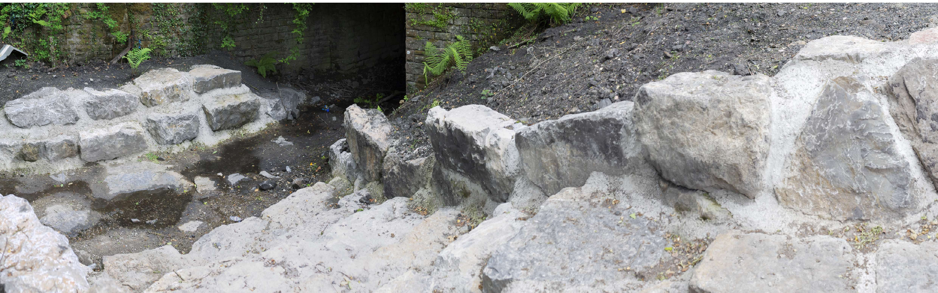
al area of the site showing the recent engineering works that have been carried out by Merthyr Council showing the construction of the boulder lined cascade close to a tunnel
