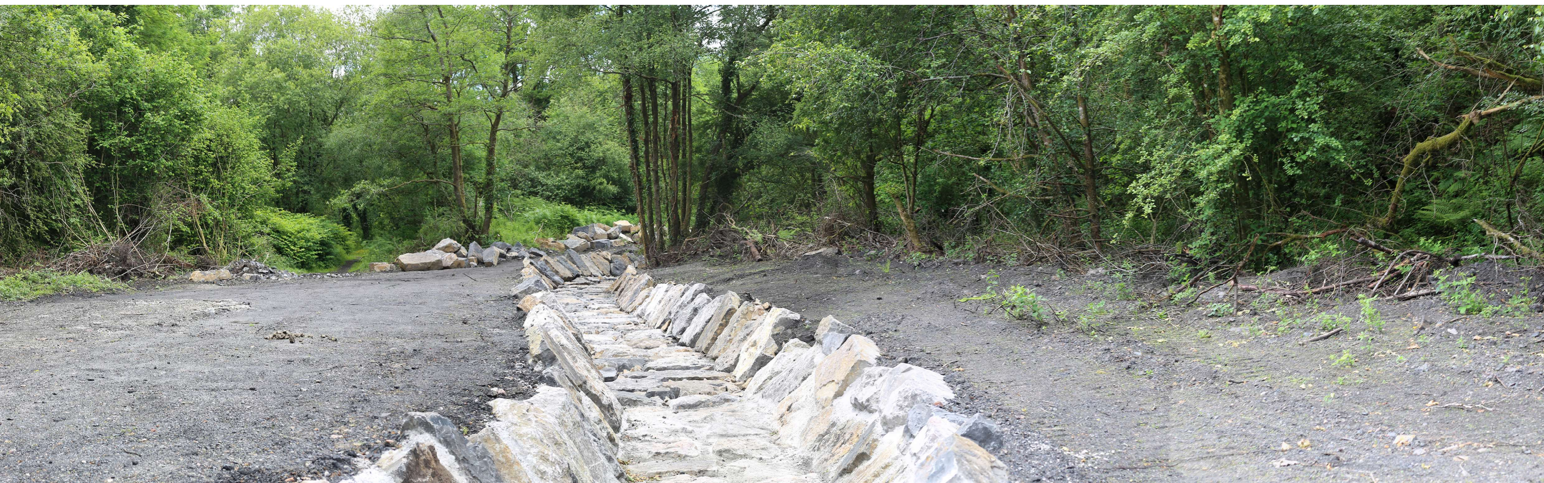
al area of the site showing the recent engineering works that have been carried out by Merthyr Council showing the construction of the boulder lined channel, the removal of some trees and the widening of the track
