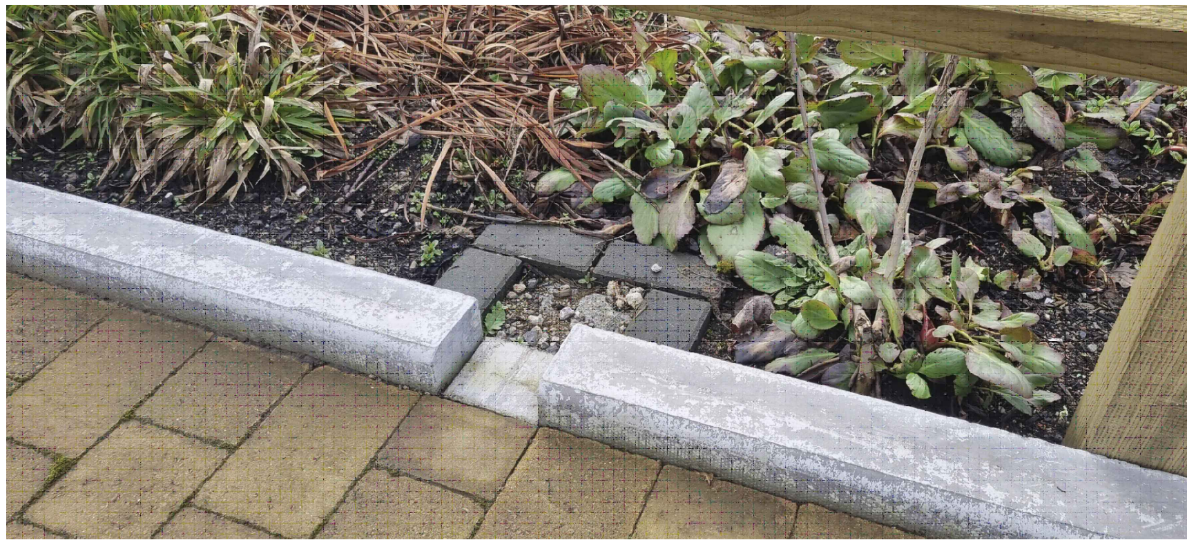
EXAMPLE OF KERB INLET TO BIORETENTION
