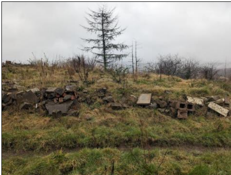
Figure 17. Concrete / stone enforced embankment (TN3, Section 10)
