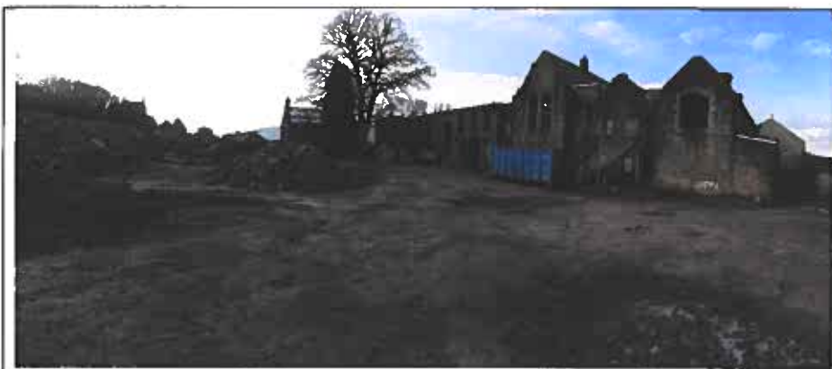
Plate 2: Panorama photograph of lower level site showing the asphalt court-yard.
