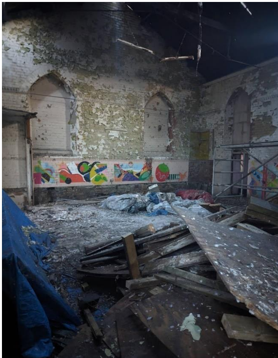
Plate 4- photograph of interior with caved in areas
