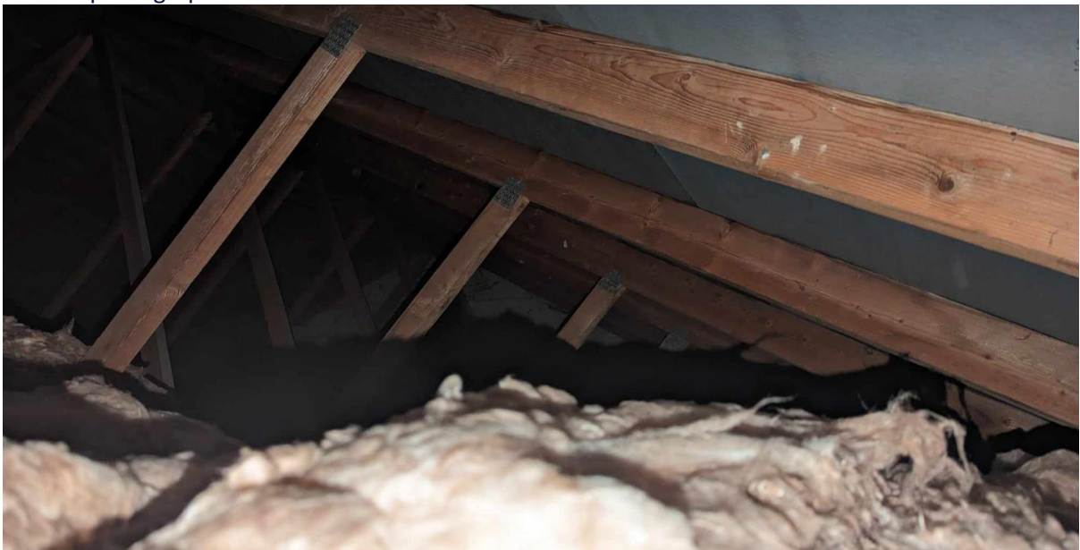
Plate 4- photograph of north western roof void
