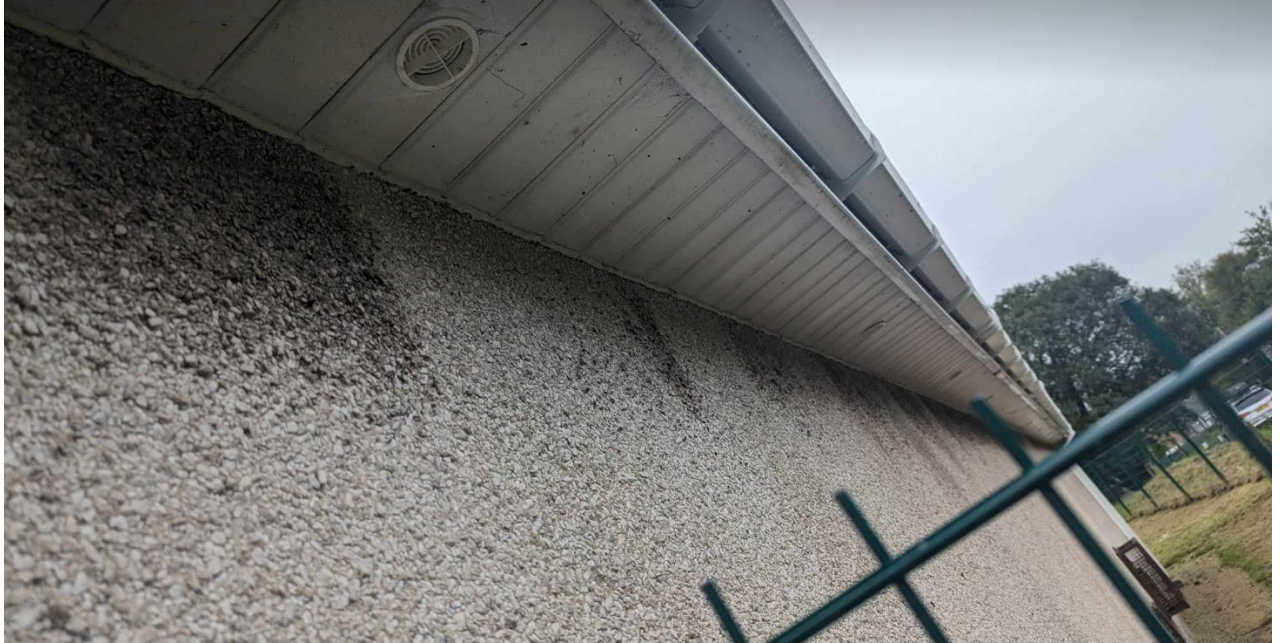
Plate 7- photograph of sealed fascias
