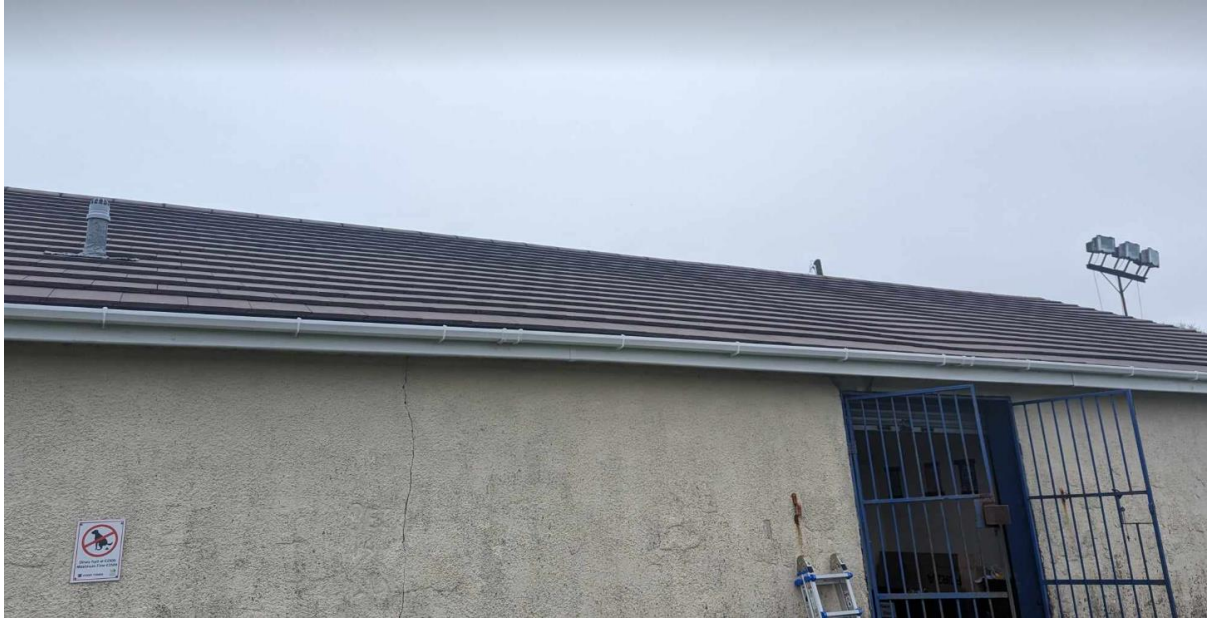
Plate 6- photograph of gable end with small gaps beneath barge boards
