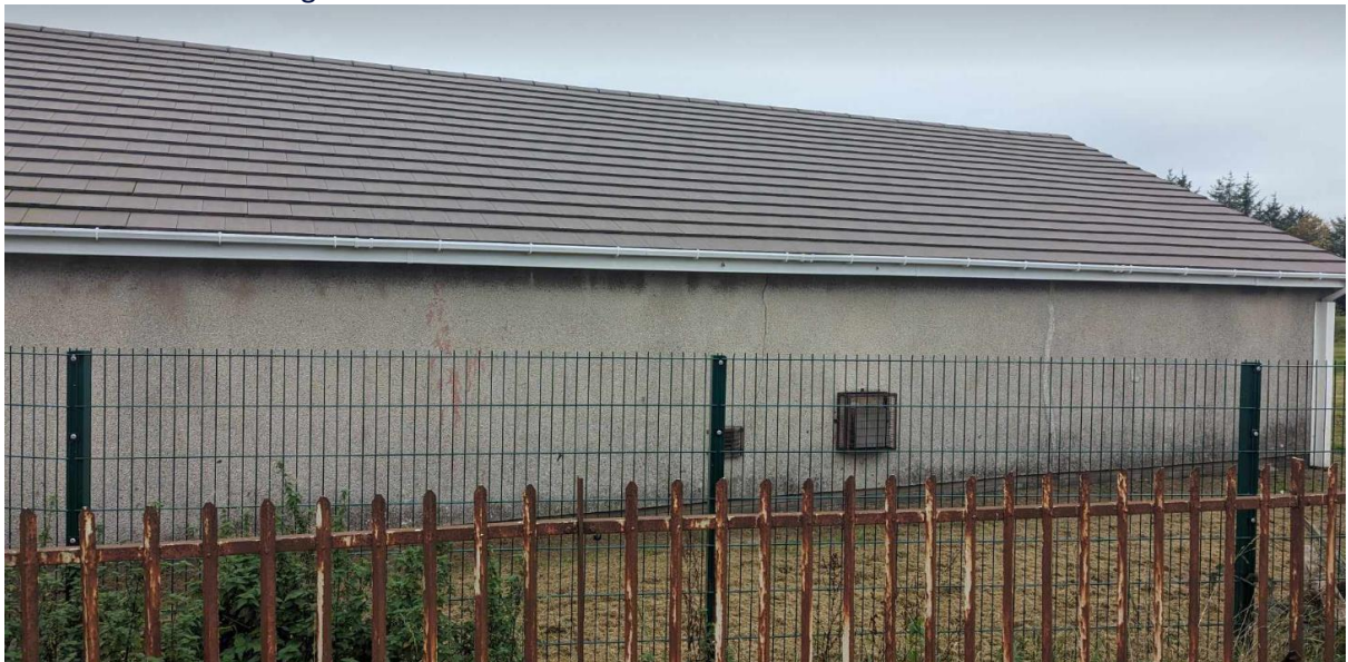
Plate 8- rear of building
