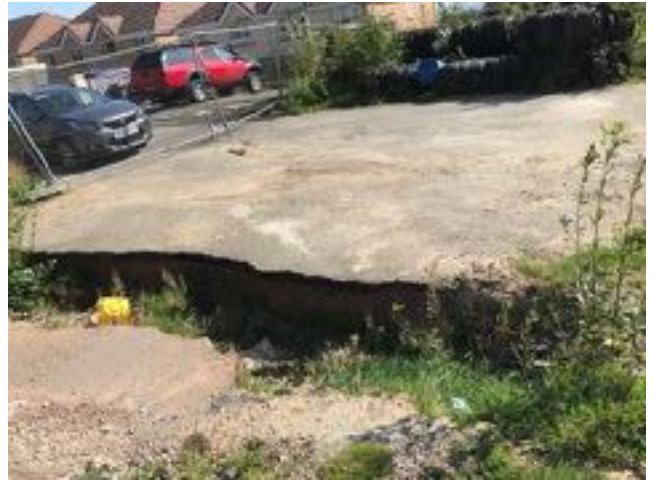
Tarmac turning area
