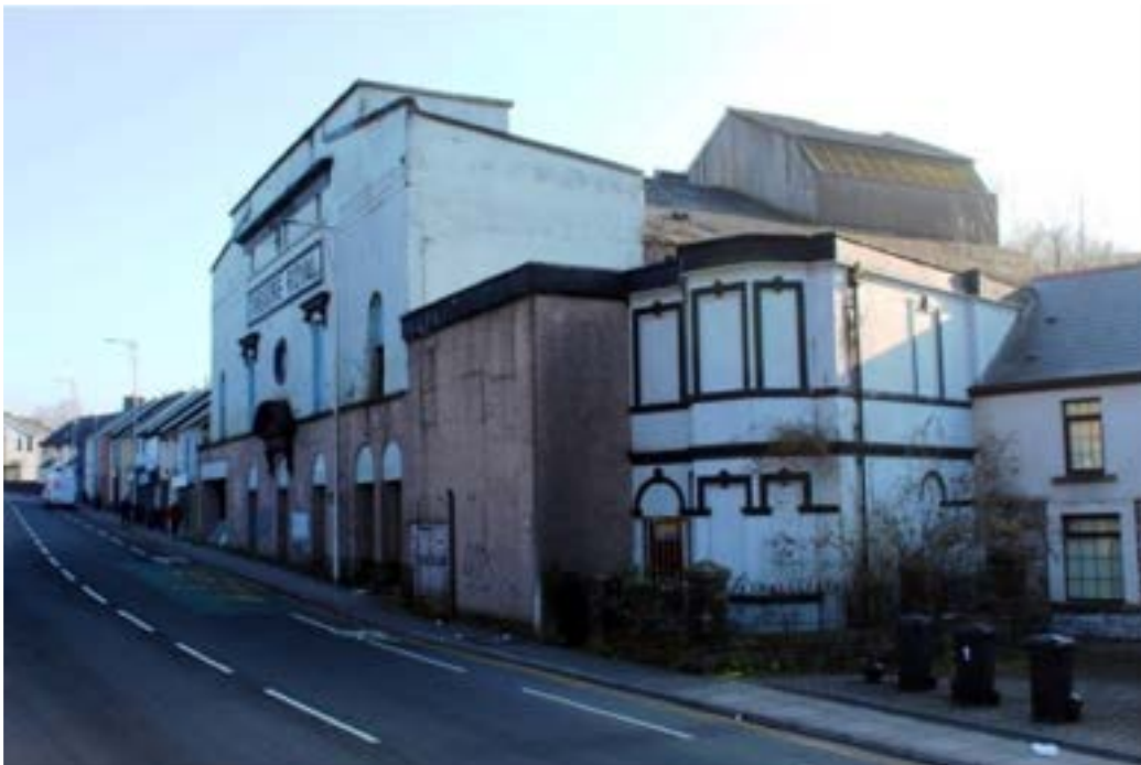
Thespian House and adjacent Theatre Royal – 2019, current condition
