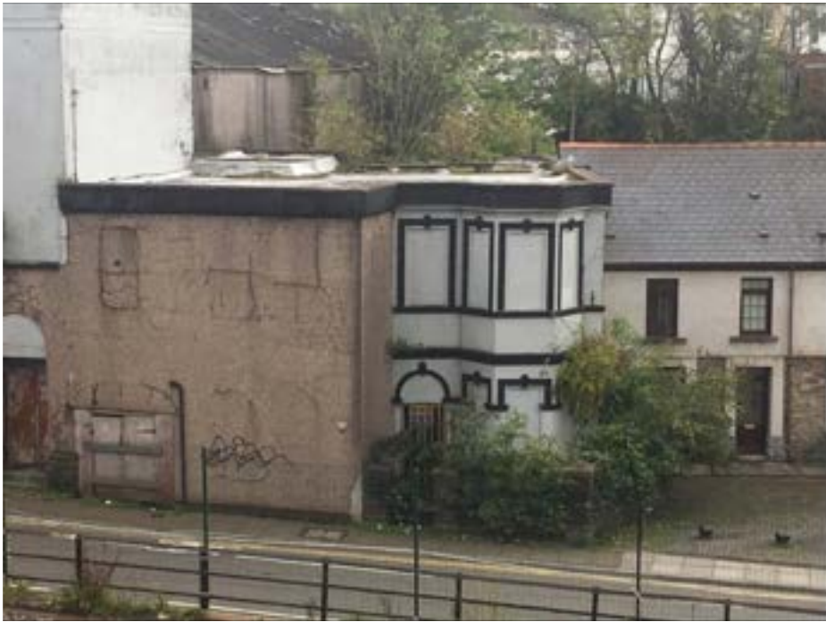
Thespian House – current condition
