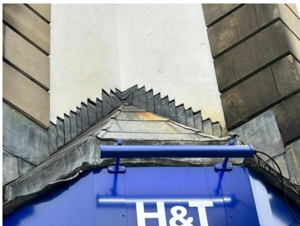
Photo 5: Lifted Lead Flashing South-East Elevation
