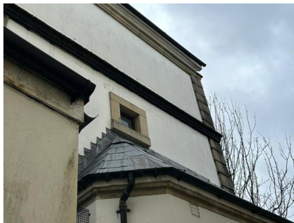
Photo 6: Lifted Lead Flashing Western Elevation
