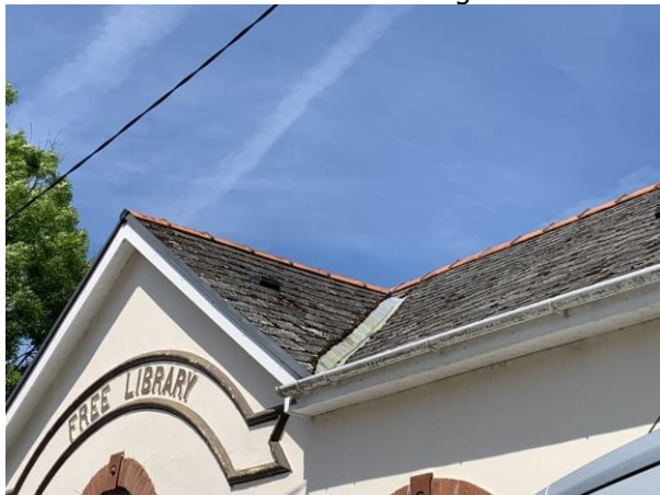
Photo 5: Roof tiles and lead flashing
