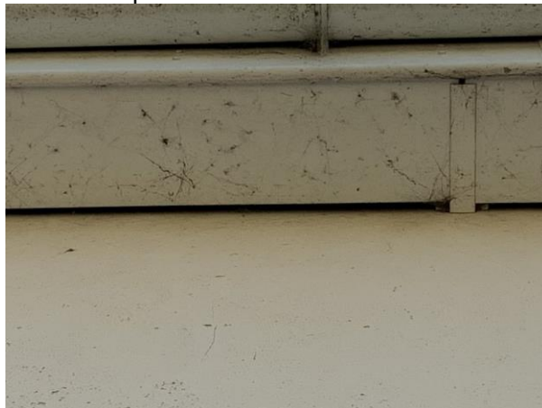
Photo 6: Gap behind uPVC soffit
