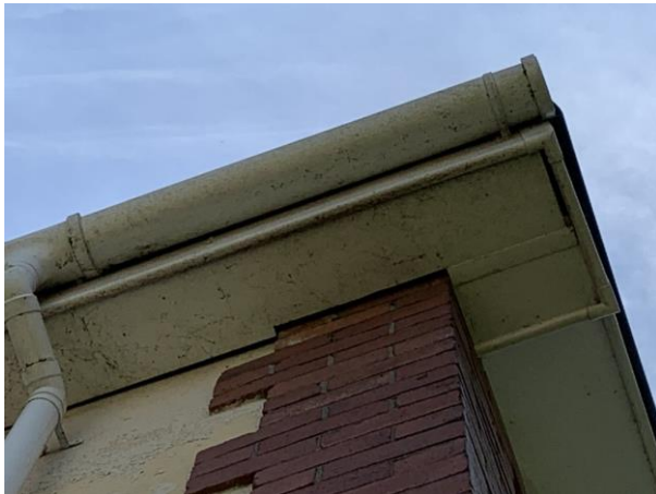
Photo 9: Gaps in Soffit on western gable end with visible apex
