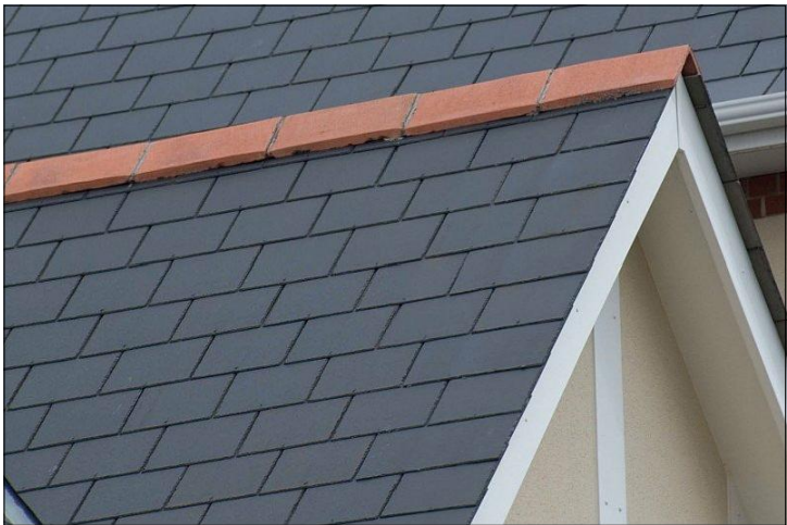
1 Marley Fibre Cement slate
