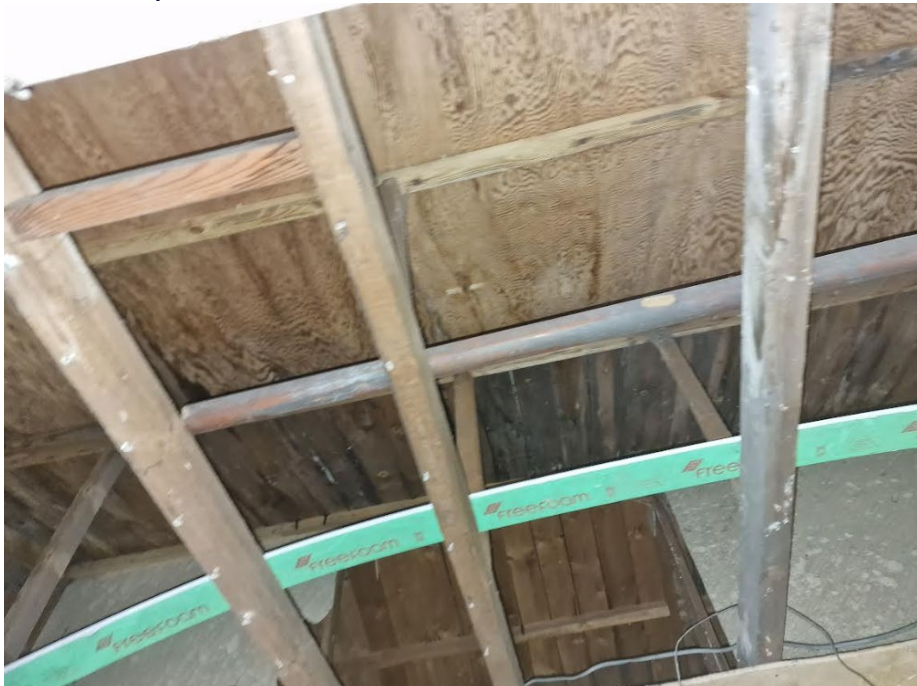
Plate 2- example of underside of cabin roof
