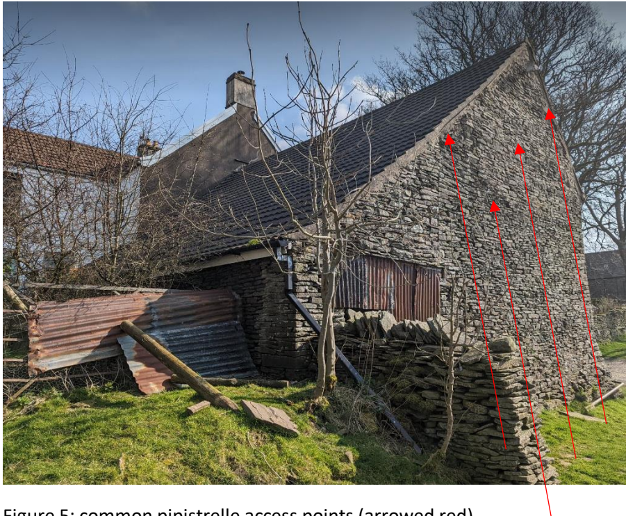
Figure 5: common pipistrelle access points (arrowed red)
