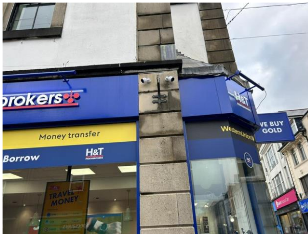
Photo 16: Shop Lighting Southern Elevation
