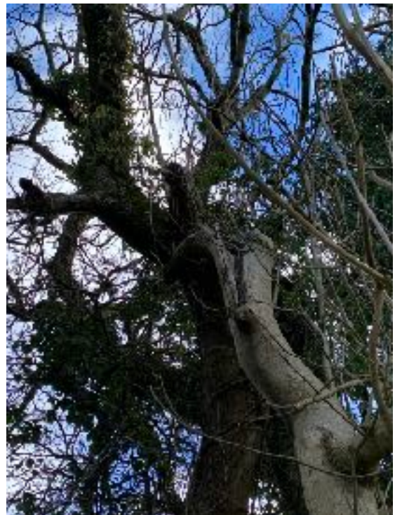
T7 West facing broken limb still attached with large crack and lifted bark.
