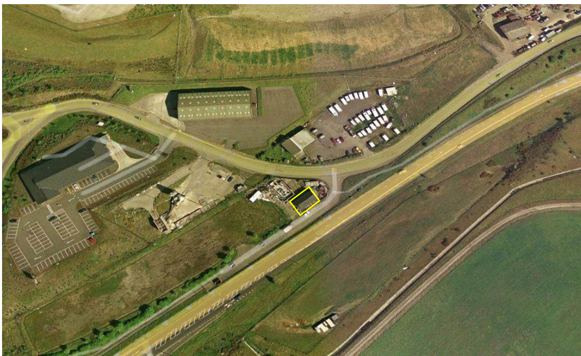
Figure 4.5 Aerial imagery of the site and surroundings in 2001.
