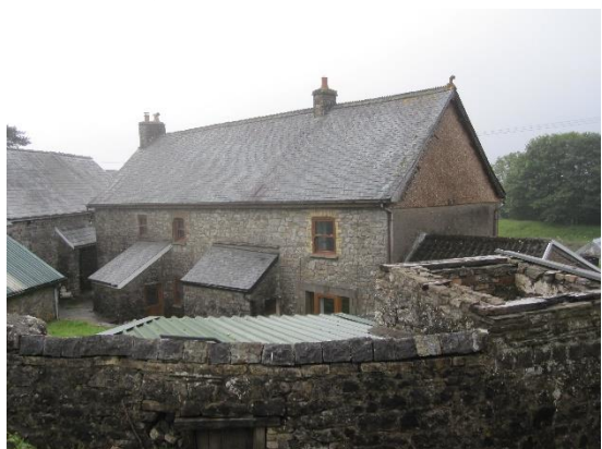
Plate 4: South-western aspect of roof, with raised or missing slates
