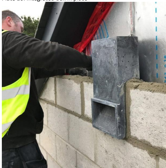
Plate 16: Integrated box in place
