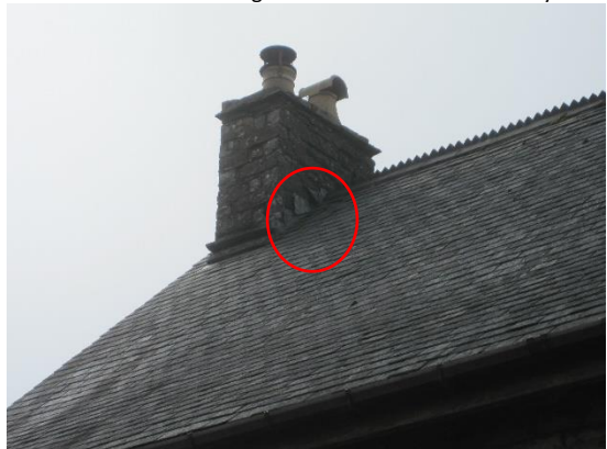
Plate 8: Lifted lead flashing around eastern most chimney
