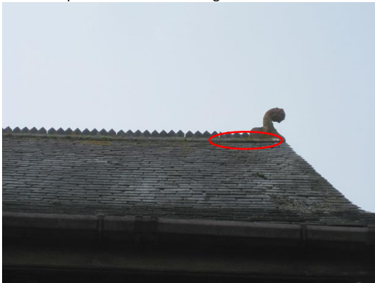
Plate 7: Gap on northern side of ridge and western end
