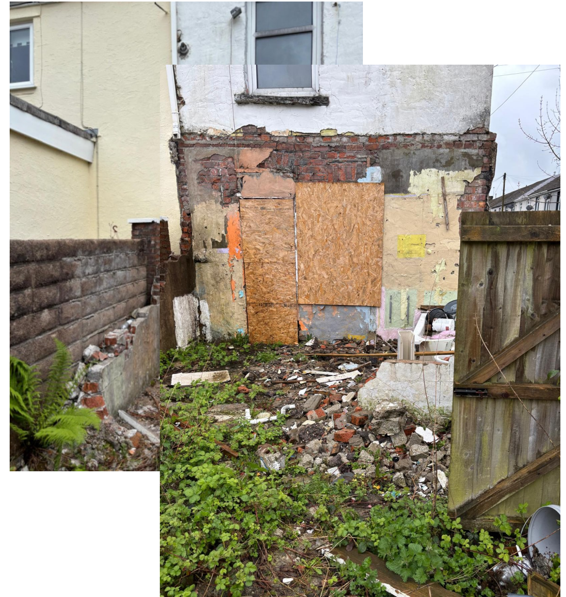
CURRENT PHOTOGRAPH OF REAR ELEVATION
