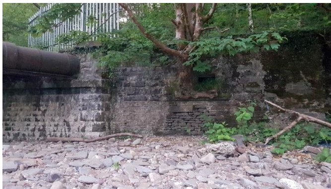
Photograph 1 Bridge showing abutment at North-west end.
