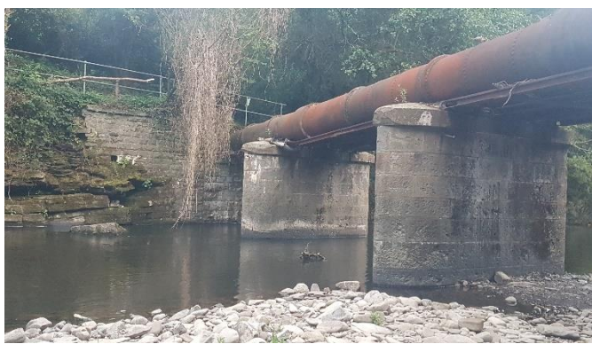
Photograph 2 Bridge showing abutment at south-east end.
