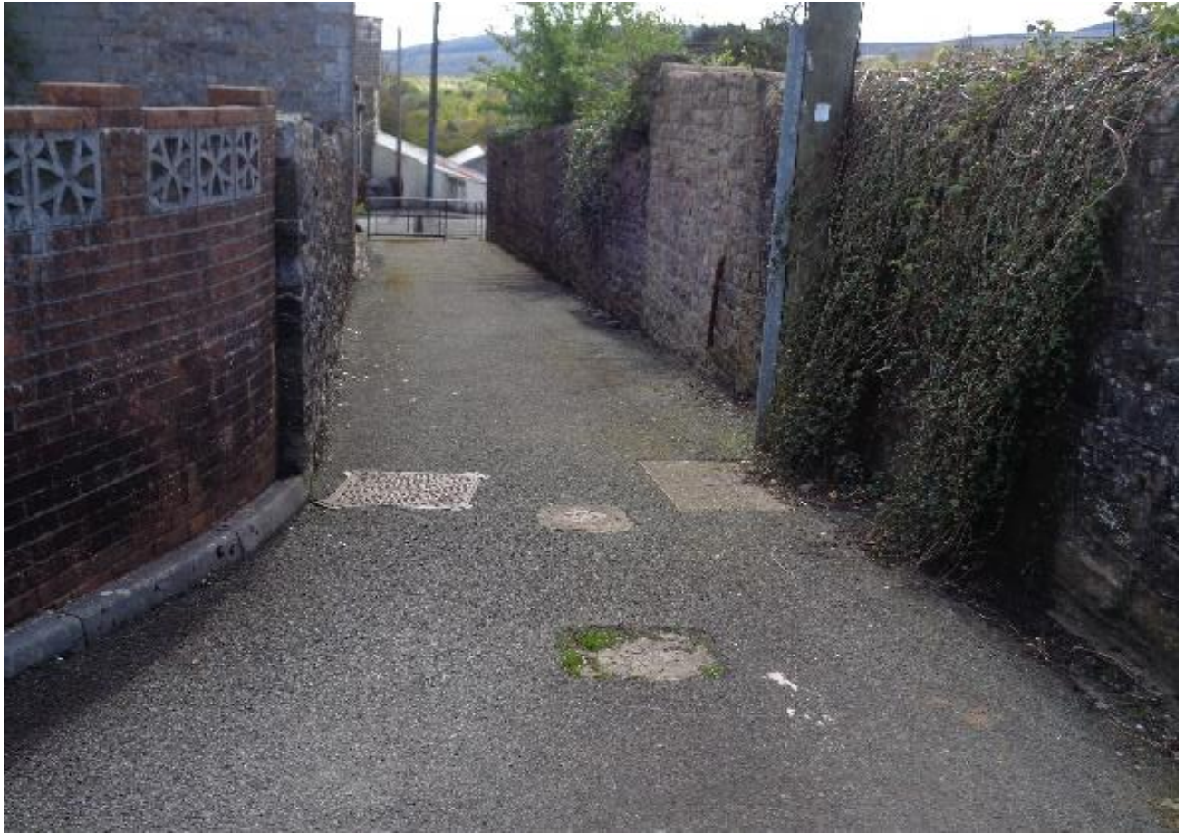
Figure 15 – Pedestrian footway on Old Church Street, facing south.
