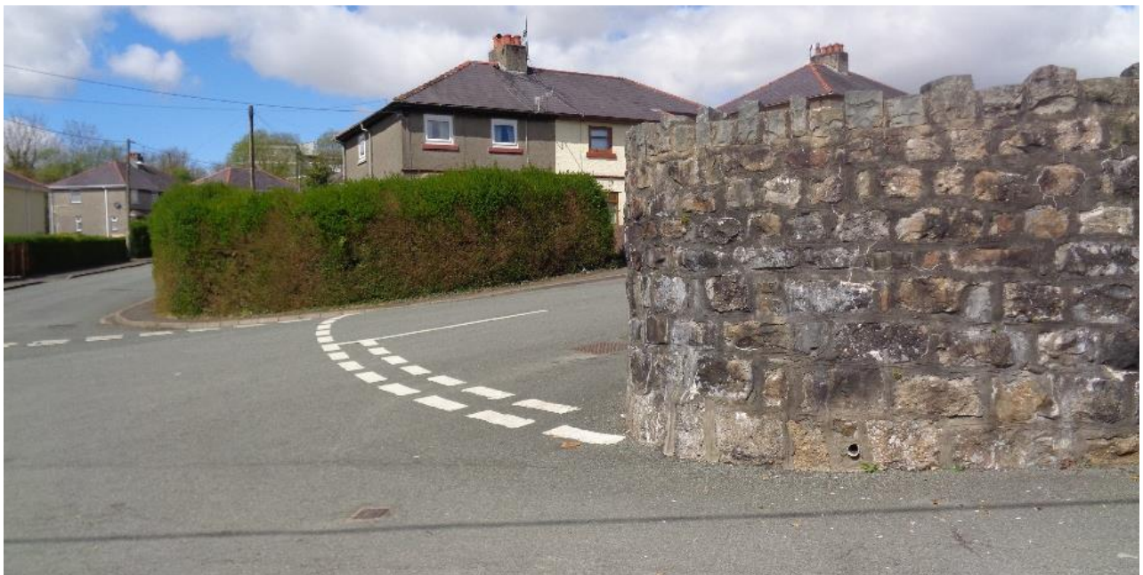
Figure 18 – Restricted visibility for movements at six-arm priority junction.
