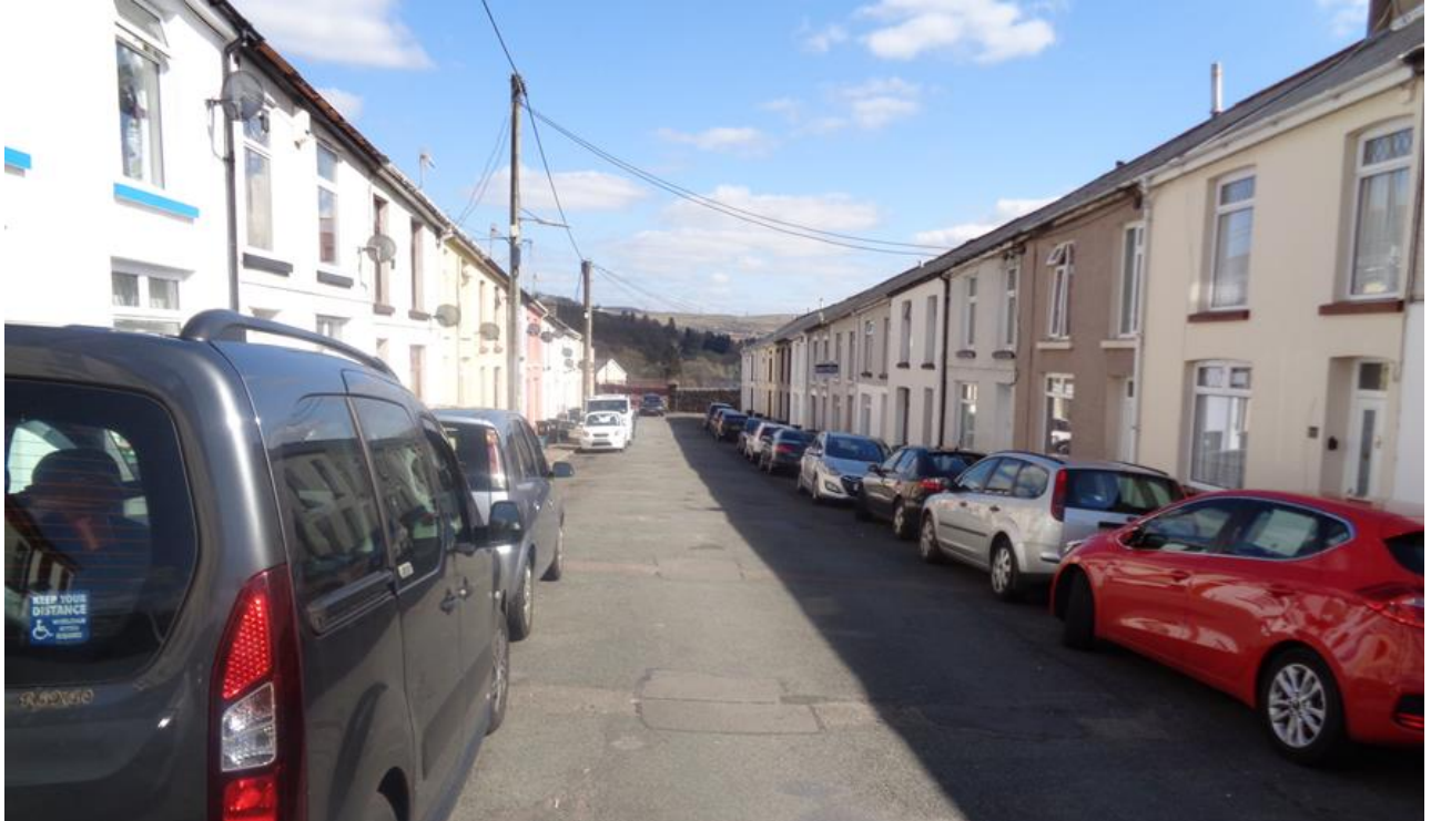
Figure 19 – South Terrace, facing south-east.
