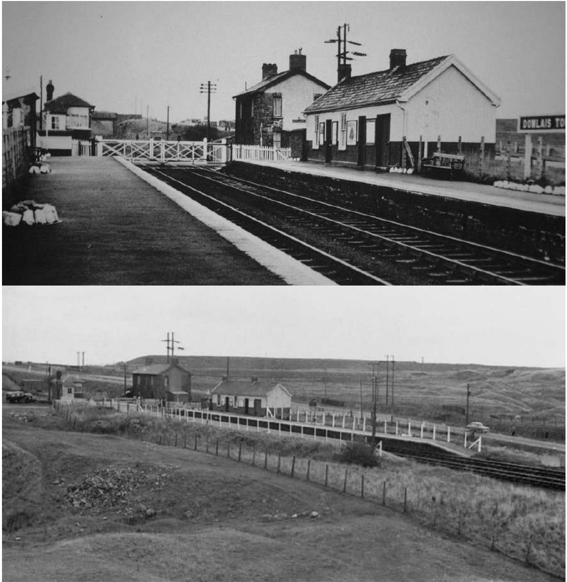
Figure 4.3 Dowlais Top Station (looking northeast), 1955 (above) and 1960s (below). Station House (northwest elevations) visible along with a station facilities building to the east and signal box to the north of the railway.
