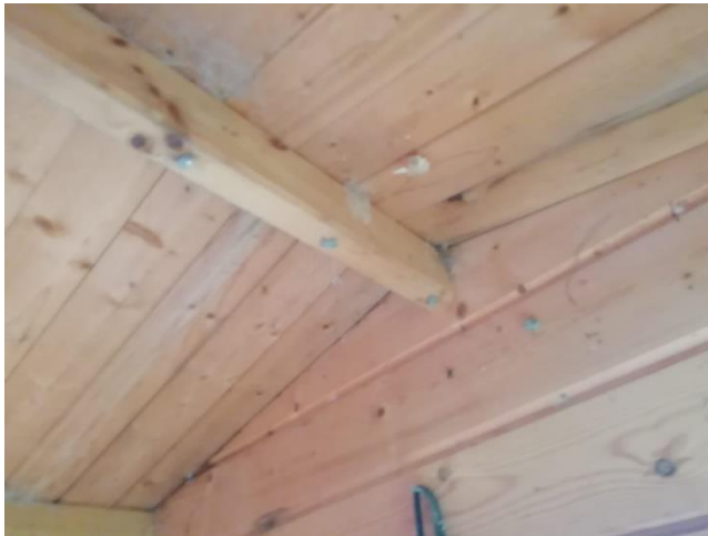
Figure 15 – Interior of most intact shed ceiling (old wasps' nest)
