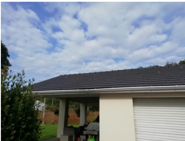
Figure 7 – View from west over northern end of garage
