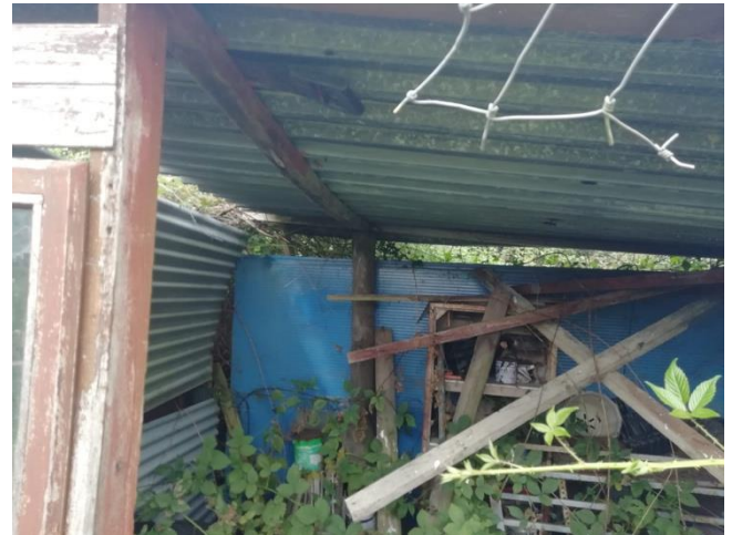
Figure 16 – Interior of second outbuilding
