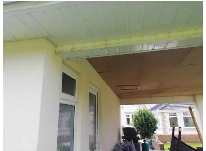
Figure 10 – Underside of sheltered area (northern section)
