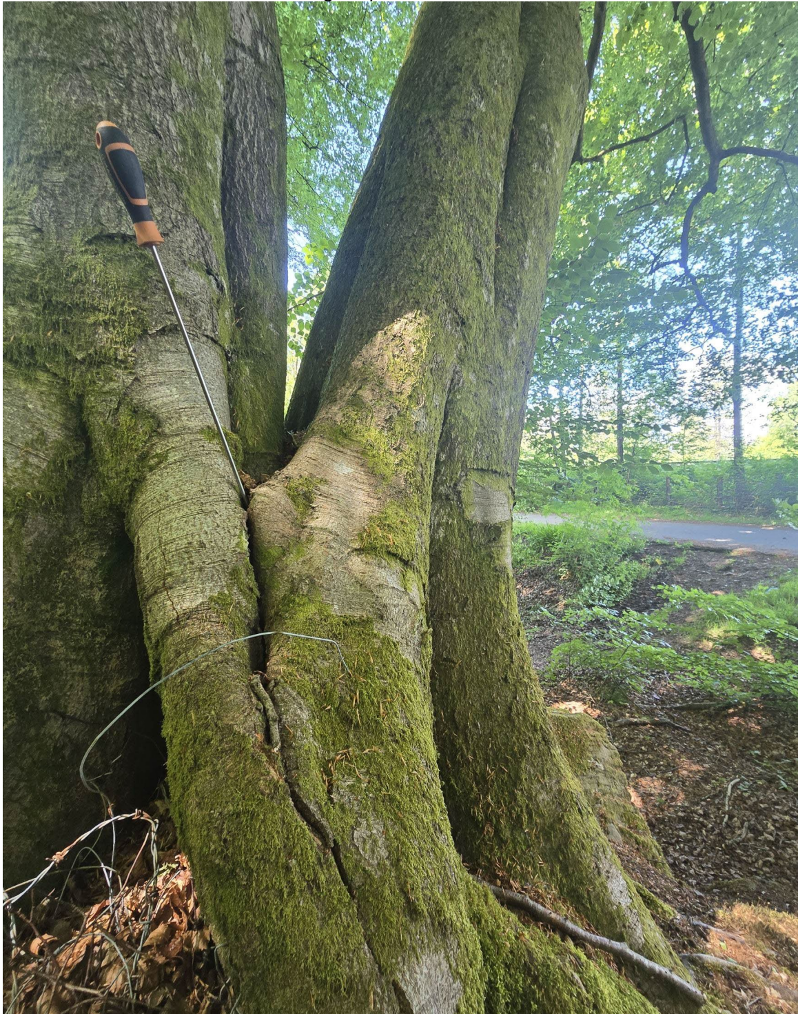
Photo I5: T32 failing compression fork observed at the base.
