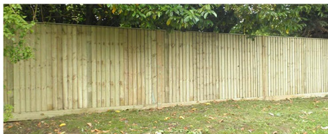
Example feather edge timber close board fence
