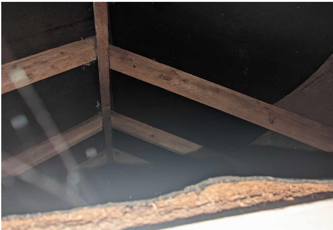
Plate 10- photograph of roof void above garage
