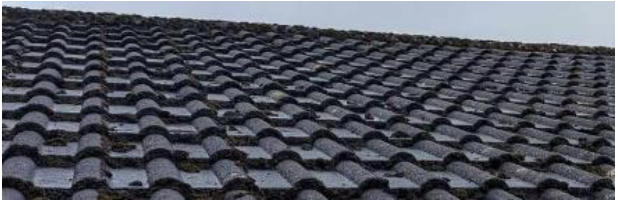
Plate 8- photograph of tight fitting tiles on garage
