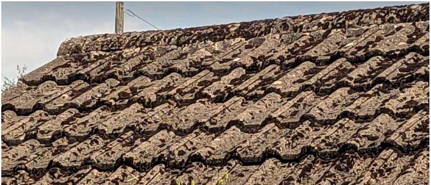
Plate 8- photograph of tight fitting tiles on garage
