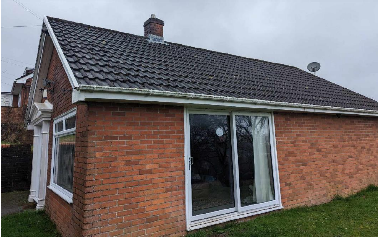
Plate 2- example of this gaps at eaves level
