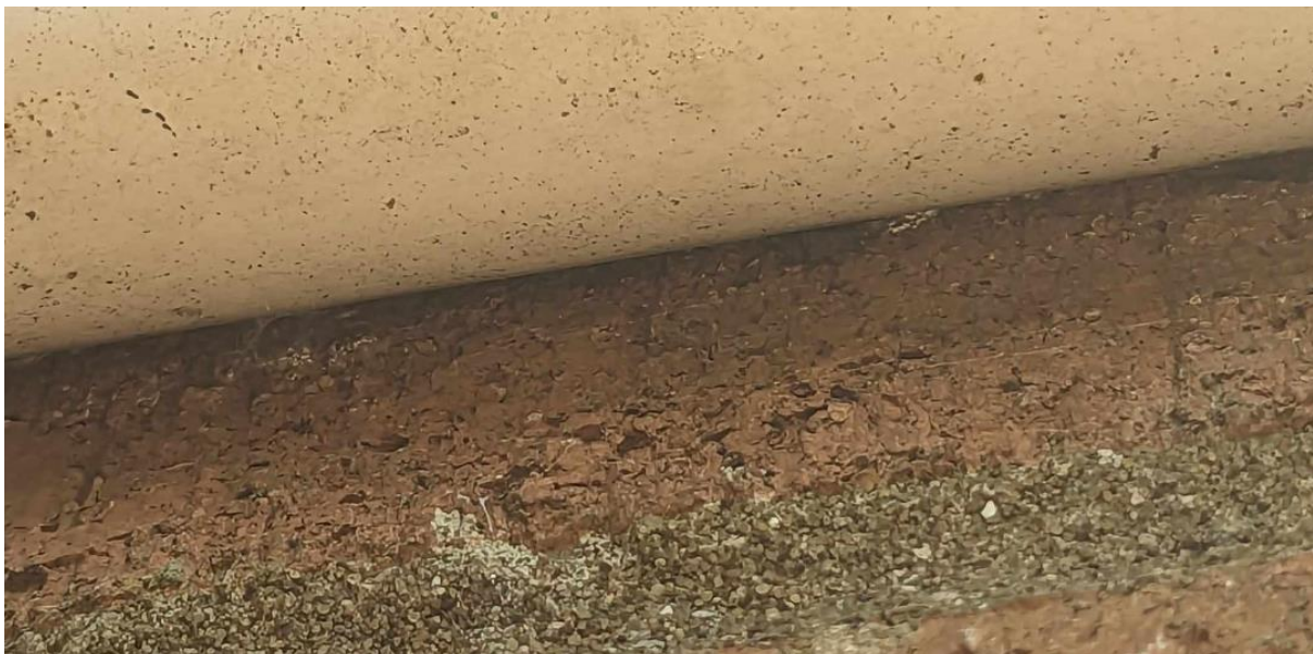
Plate 14- Close up of gap between wall and uPVC of garage (showing very little access space)
