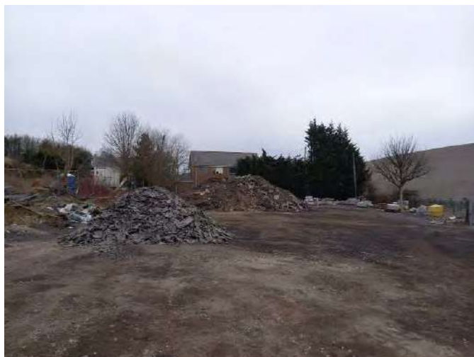
View from east of site looking north.
