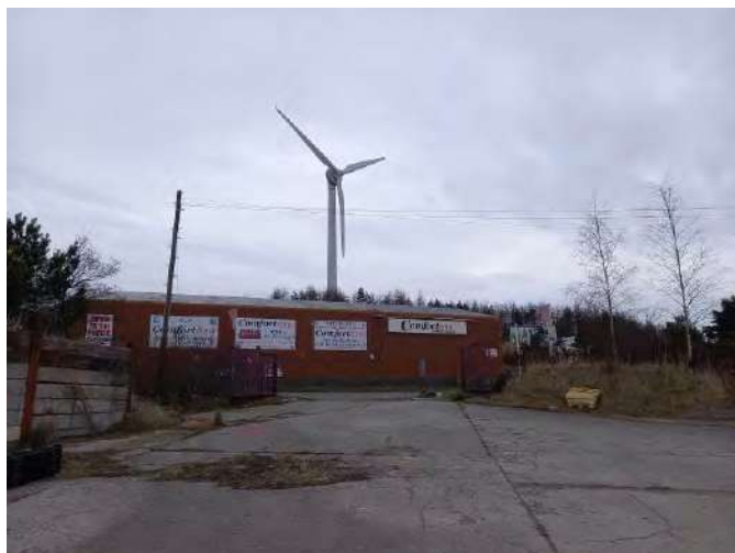
View from centre of site looking north.
