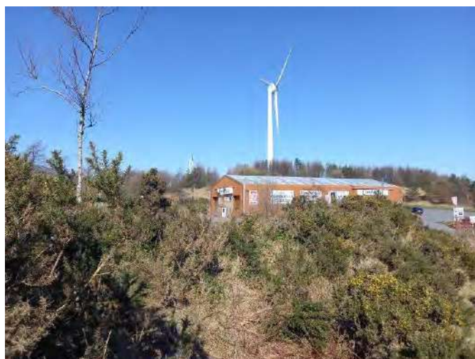
View from top of western bund looking north.
