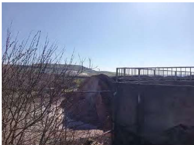
View from south east of site looking south east.
