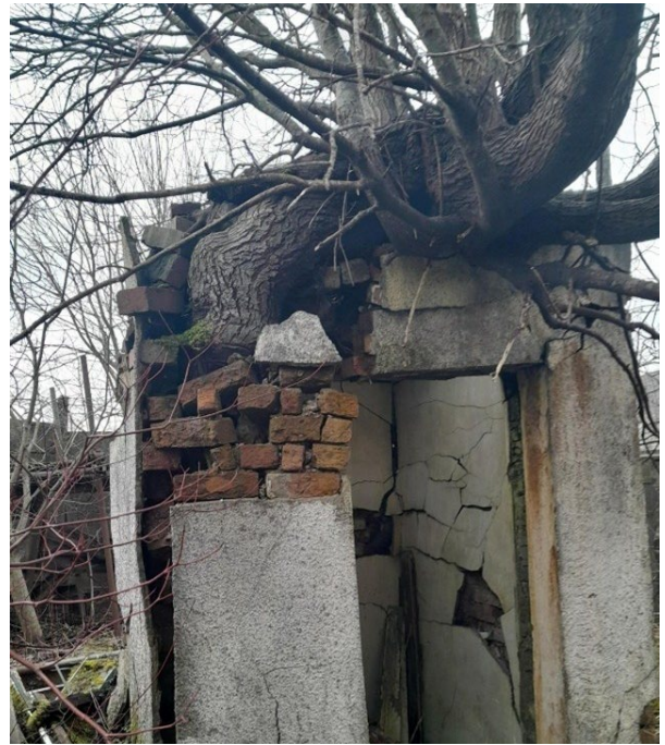
Image EDP A3.8: Built Structure B2 with willow growing through.
