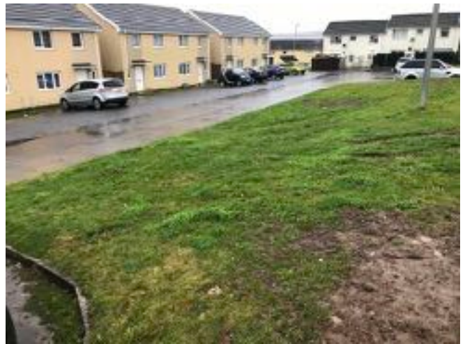
Looking south west
