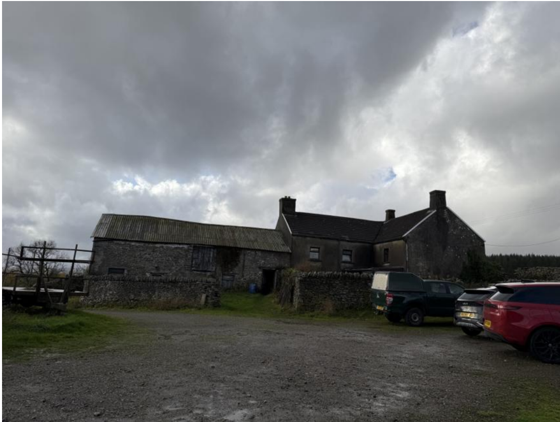
Figure 1: Photograph of existing farmhouse
