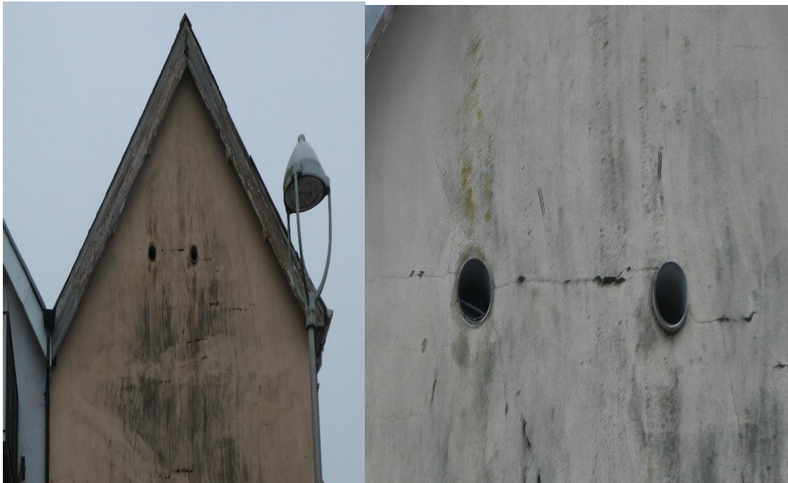
Plate 11 – View of neighbouring property to southern end rear wall with openings to loft
