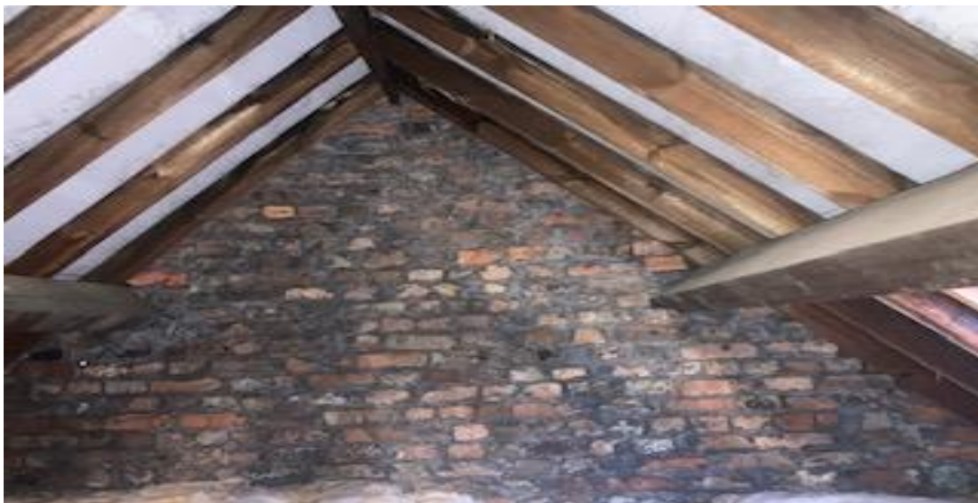
Plate 4 – Internal views of eastern wall in loft
