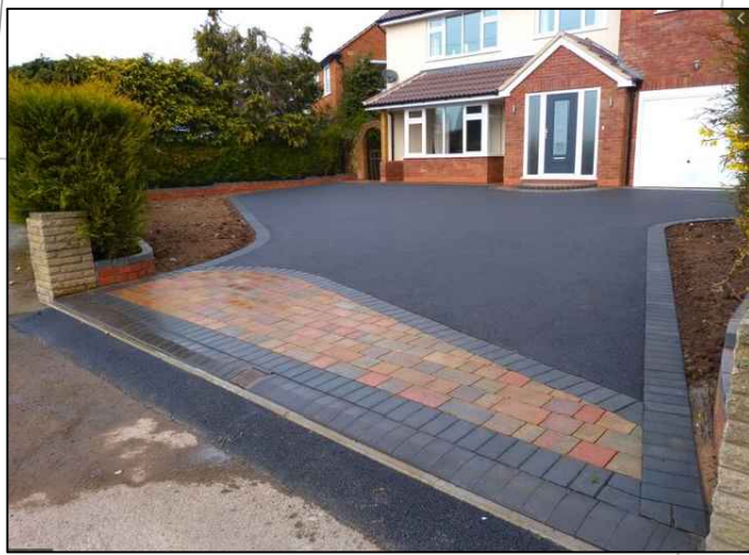
TYPICAL IMAGE OF A POROUS ASPHALT DRIVEWAY
