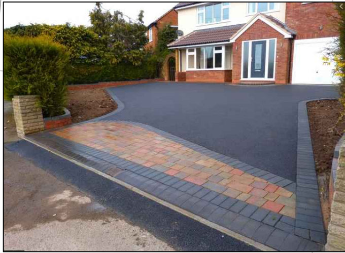
TYPICAL IMAGE OF A POROUS ASPHALT DRIVEWAY
