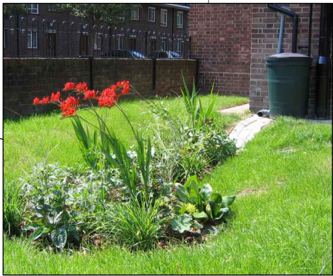
TYPICAL IMAGE OF A BIORETENTION RAINGARDEN
